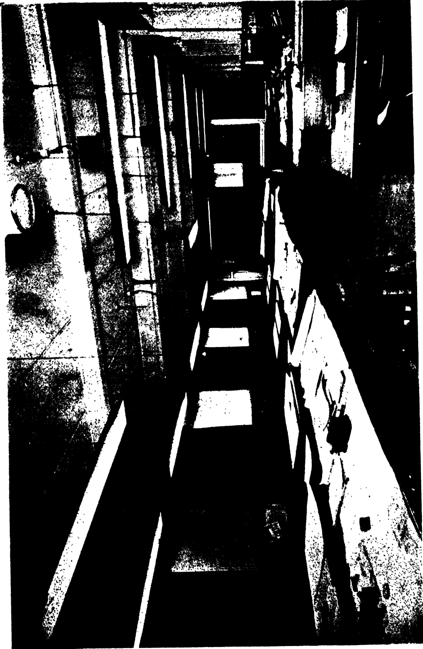
Fig. 39.—DRAWING OFFICE LIGHTING. ( Reflectors placed mutually at right-angles help to reduce shadow, especially in a small installation.)
