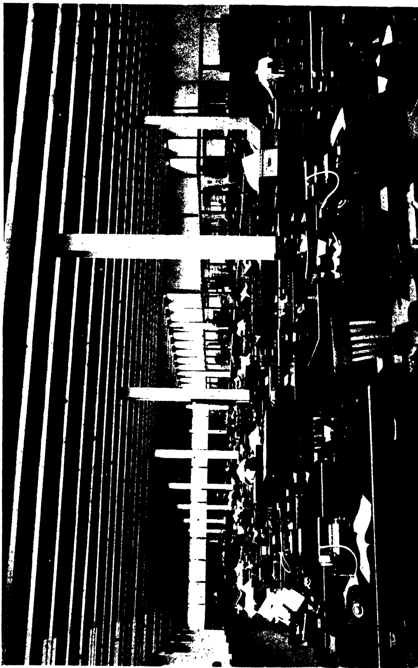
Fig. 65. —TROFFERS SPECIALLY DESIGNED TO PRESENT LOW-BRIGHTNESS SURFACES AT NORMAL ANGLES OF VIEW. (Louvred aluminium reflectors of modified parabolic section. Spacing, 4 ft. Note short sections at left hand end of each third main troffer; these compensate for light lost through windows.)
