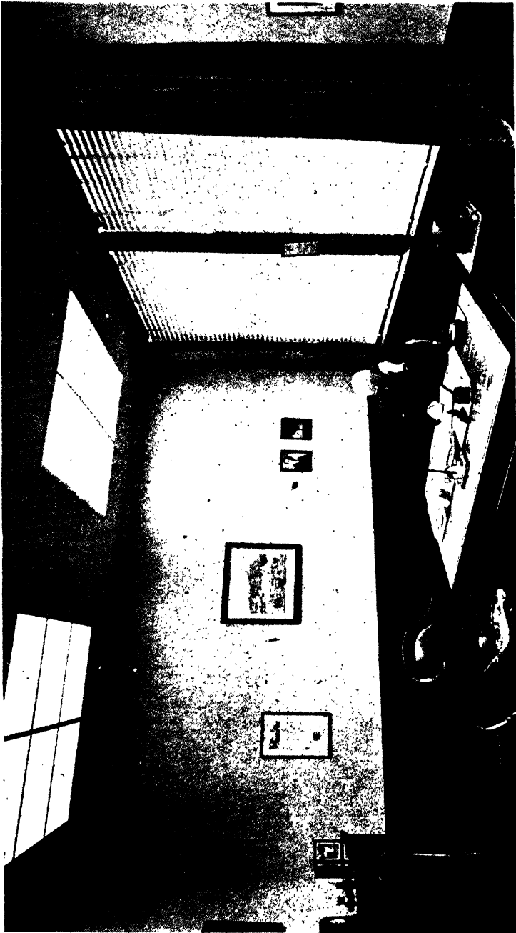
Fig. 63. —THE ILLUMINATION IN THIS 16 FT. BY 15 FT. OFFICE IS ALMOST 100 FOOTCANDLES, PROVIDED BY FOUR RECESSED COFFERS CLOSED BY DIFFUSING GLASS. EACH COFFER CONTAINS A TOTAL OF 400 WATTS OF FLUORESCENT LAMPS.
