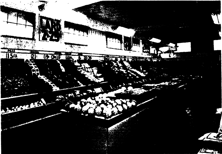
Fig. 53. —THE ROW OF SEMI-CYLINDRICAL FITTINGS CONCENTRATES ATTENTION ON THE MERCHANDISE BY LIGHTING THEM TO A HIGHER BRIGHTNESS THAN THEIR SURROUNDINGS.
