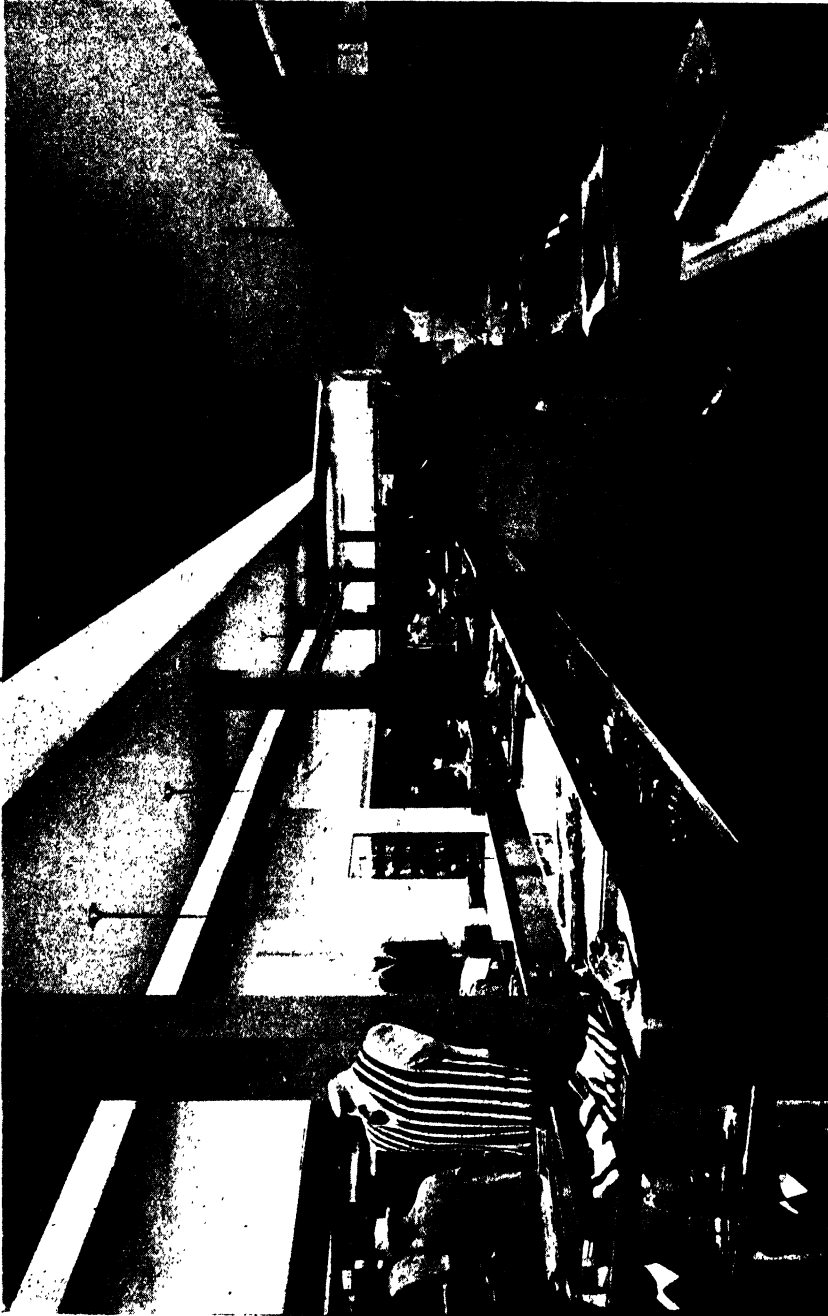
Fig. 54.—120 FOOTCANDLES ILLUMINATION—ALMOST DAYLIGHT EASE OF SEEING. (Note the supplementary indirect lighting by suspended trough fittings, the silhouetted sign over the wall case, and the almost complete absence of shadow.)
