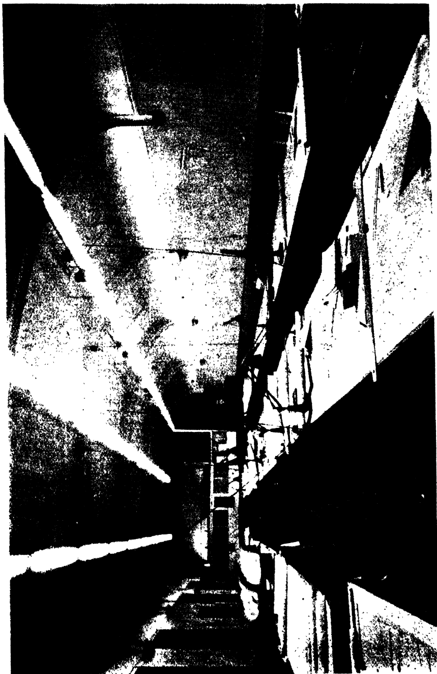
Fig. 40. A DRAWING OFFICE LIT BY FLUORESCENT LAMPS IN CONTINUOUS TROUGH REFLECTORS.
