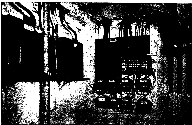
Fig. 15. Old Method of Installing Meters
