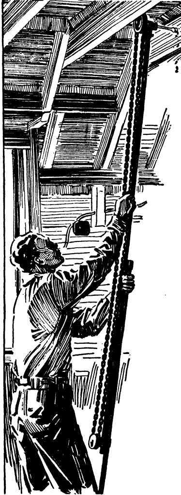
Fig. 9. Using a Joist Boring Machine Courtesy of Greenlee Tool Co., Rockford, Ill.
