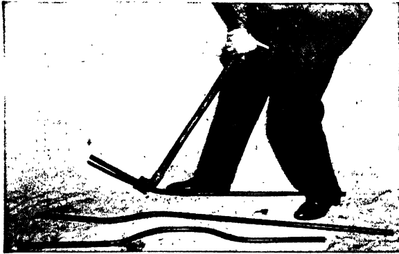
Fig. 24. Bending Conduit with Hickey. Note Saddle Bend and Offset in Conduit in the Foreground
