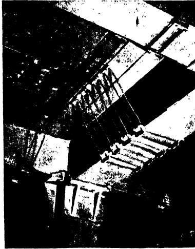
Fig. 24. Incorrect Method of Crossover Note that flexible tubing is drawn over outside in place of inside conductors.
