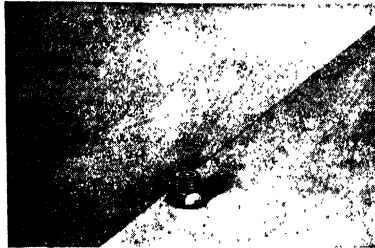
Type CCT Self-Threading Connector Installed and Ready to Continue Conduit with Rigid Threaded Connection
