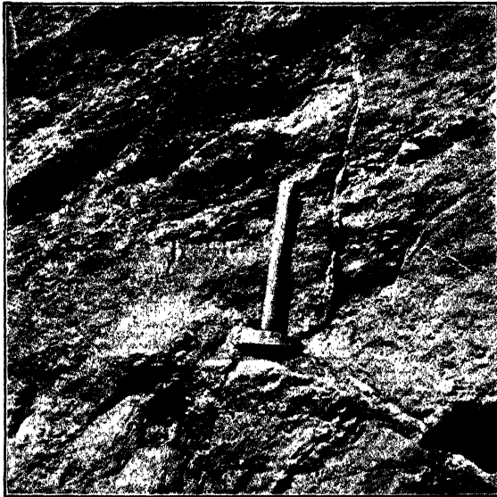
FIG. 211. — Soft conglomerate with gypsum seams. Foundation rock of part of the St. Francis dam. (H. Ries, photo.)
