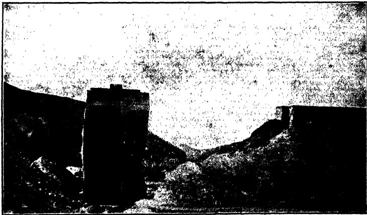
FIG. 212. — St. Francis dam after its failure. Rock on left schist, and on right soft conglomerate. The two join along a fault on slope just to right of standing section. Dam 275 feet high. (H. Ries, photo.)
