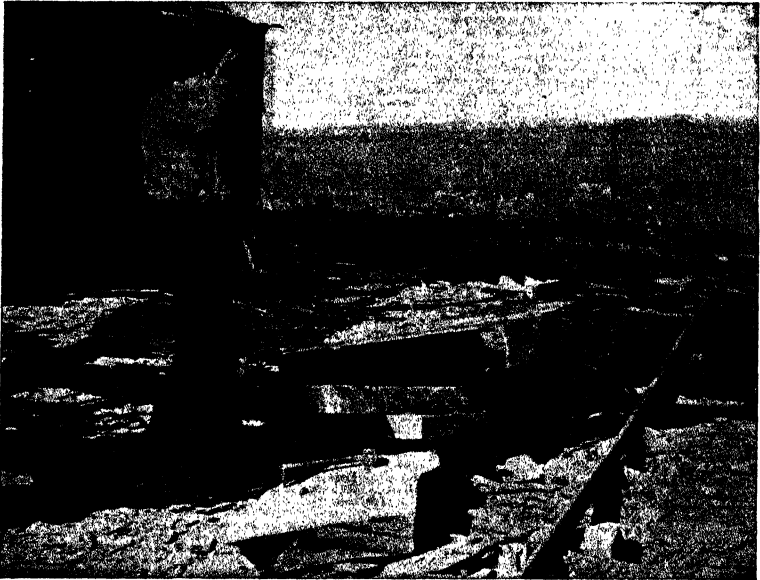
PLATE LXXIII, FIG. 1. — Sculping slate. The slab has been broken along the grain, and as the one piece dropped, it broke along the cleavage. (H. Ries, photo.)
