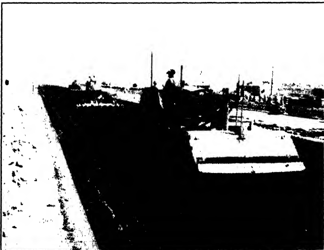
Courtesy Portland Cement Association
