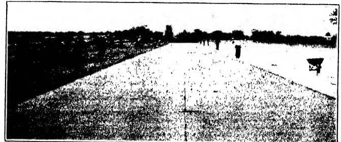
Courtesy Portland Cement Association
