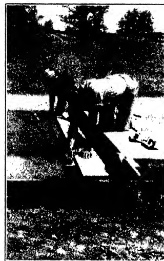
Courtesy Portland Cement Association
