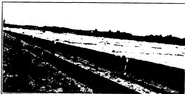
Courtesy Portland Cement Association
