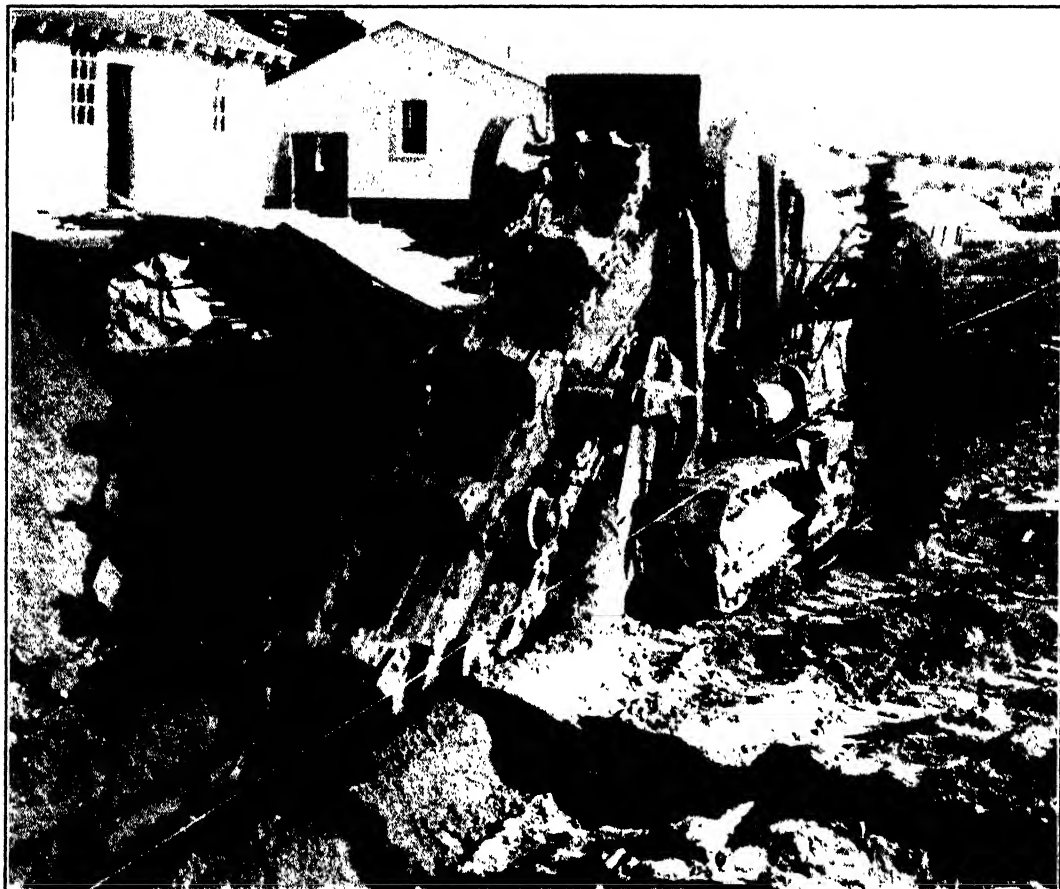
FIG. 239. Trencher operating to line and grade.
