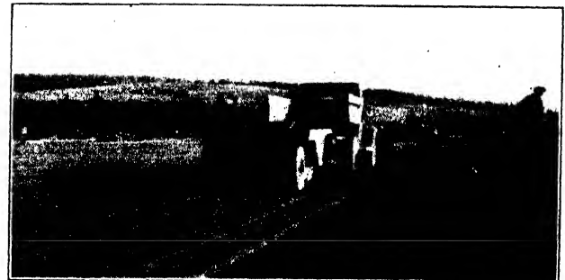
Courtesy Portland Cement Association
