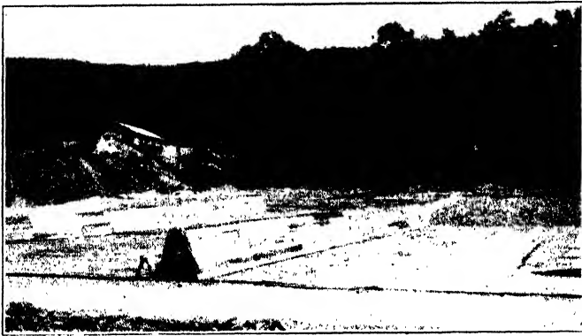
Courtesy Portland Cement Association
