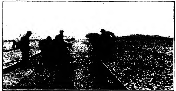
FIG. 108. Spreading the stone base.
