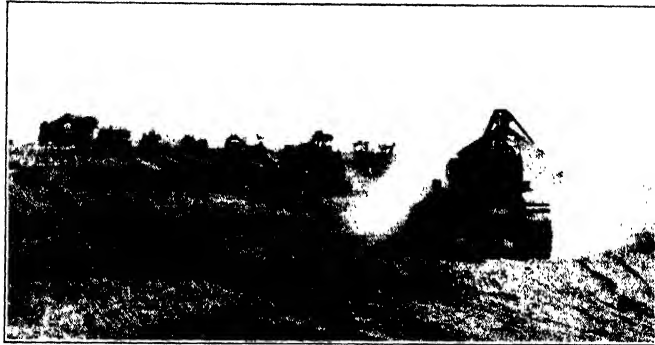
FIG. 246. LeTourneau carry-all scrapers being used on general leveling and cleaning up.
