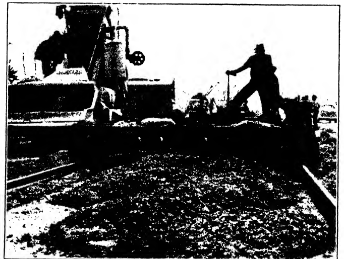
Courtesy Portland Cement Association
