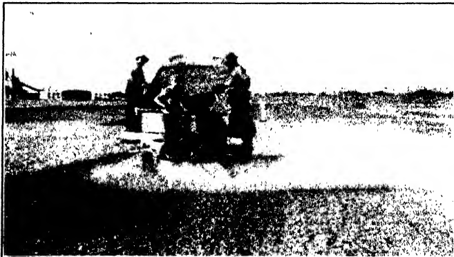
FIG. 111. Filling the voids on the surface.
