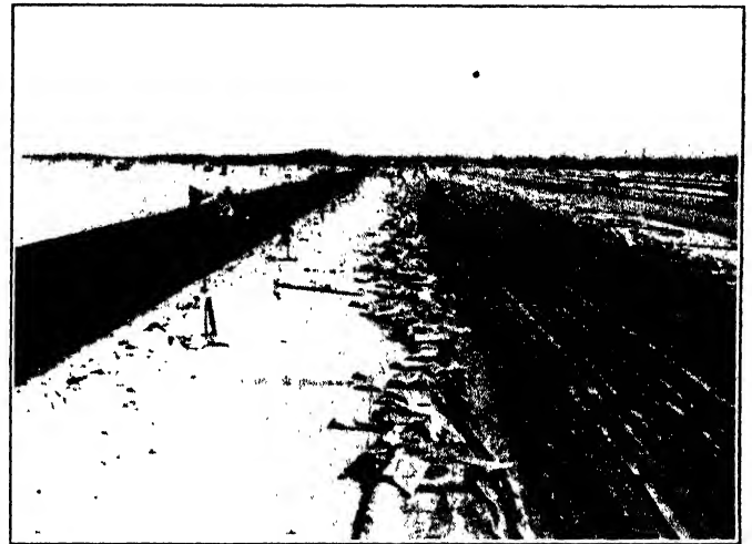
Courtesy Portland Cement Association
