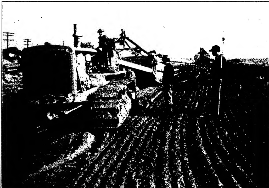
FIG. 236. Compacting and mixing.
