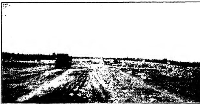
FIG. 23. An airport is a huge area, involving anywhere from 100,000 to 1,000,000 square yards of paving. The first step is to grade the field to proper cross section.
