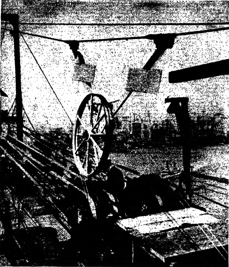
FIG. 40.—Strand shoes and spinning carriage, San Francisco Bay Bridge. (Courtesy of the American Bridge Co.)
