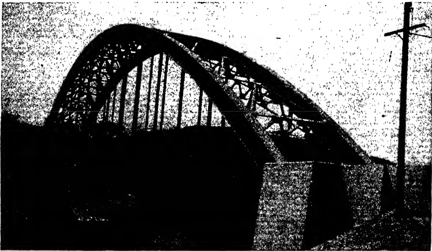
FIG. 27.—Orford-Fairlee Bridge, over Connecticut River.
