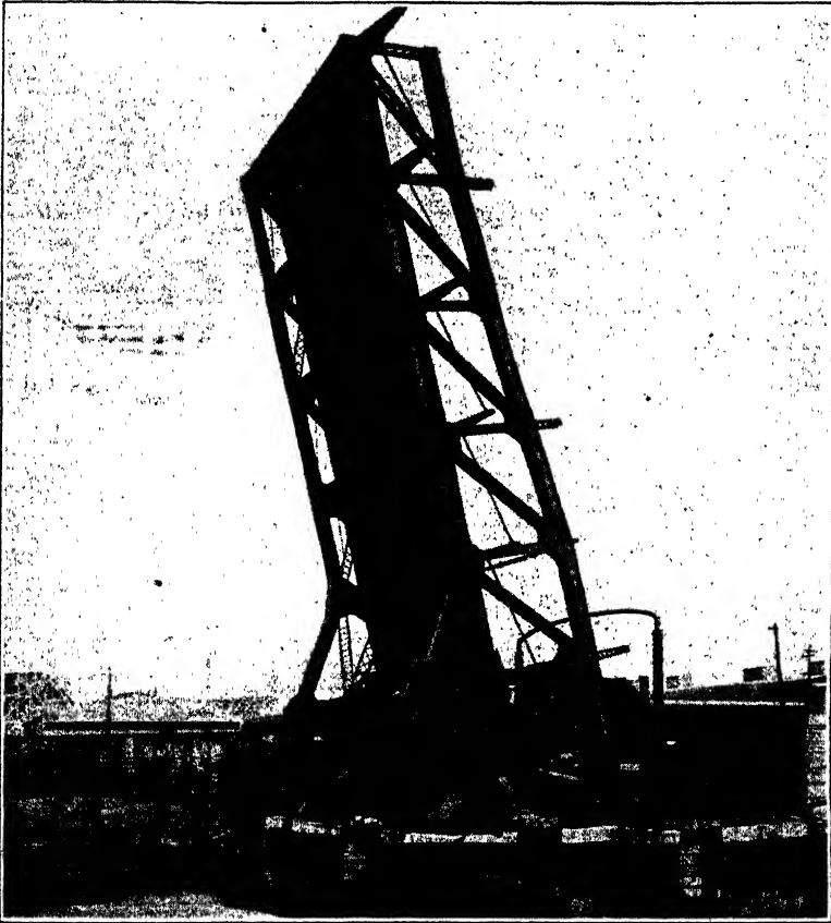
FIG. 31.—East abutment, Belmont Avenue Bridge, Chicago, Feb. 1, 1916.
