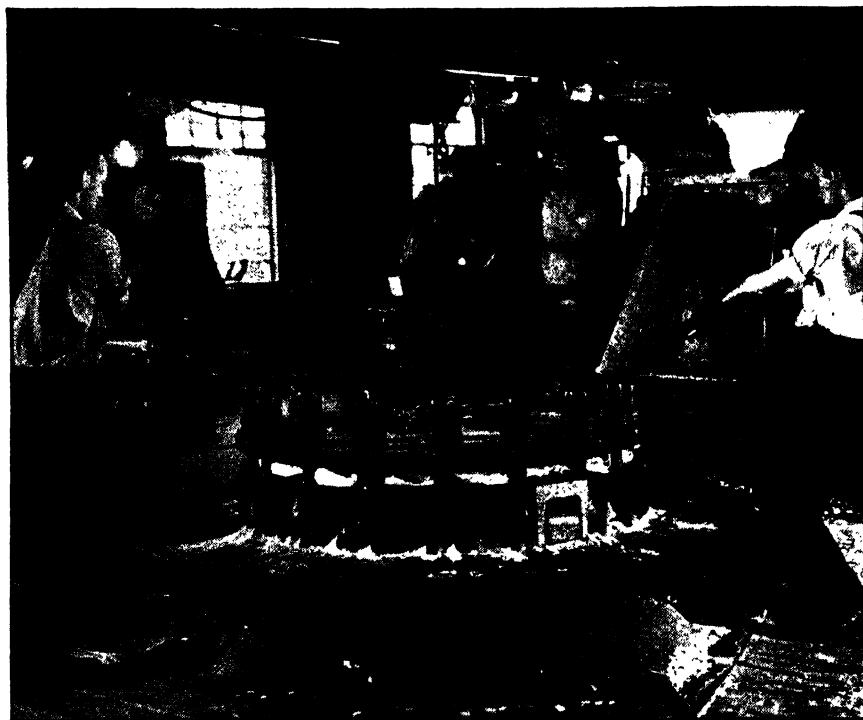
FIG. 2. Bolting on Cover of Charged Digester.†
