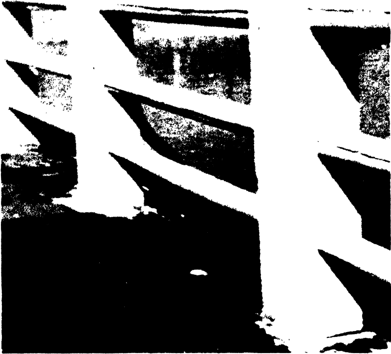
Figure 6.64a. Flash marks produced by thermal radiation on asphalt of bridge. Where the railings served as a protection from the radiation, there were no marks. The length and direction of the "shadows" indicate the point of the bomb explosion.
