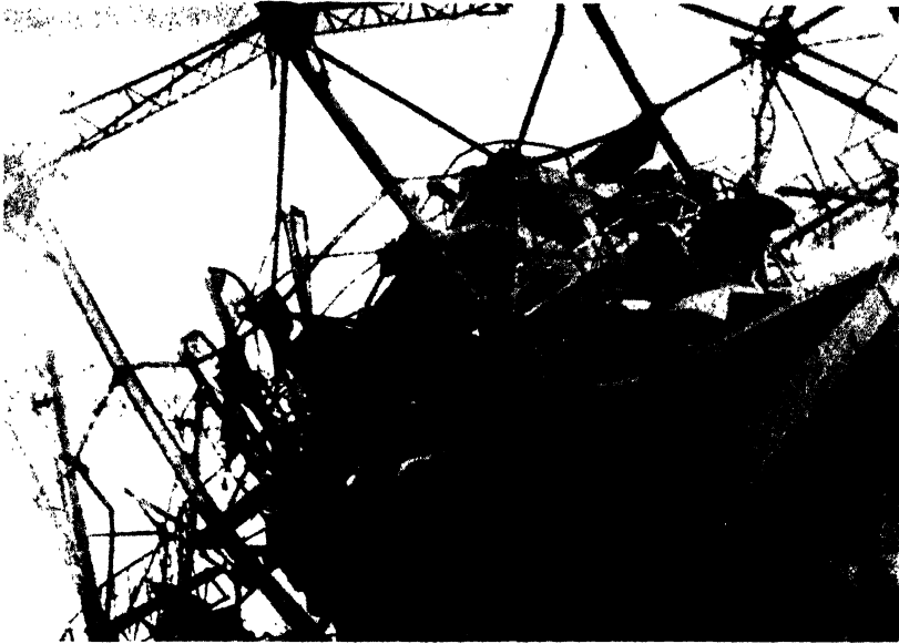
Figure 5.69b. Destroyed gas holder, 3,200 feet from ground zero.
