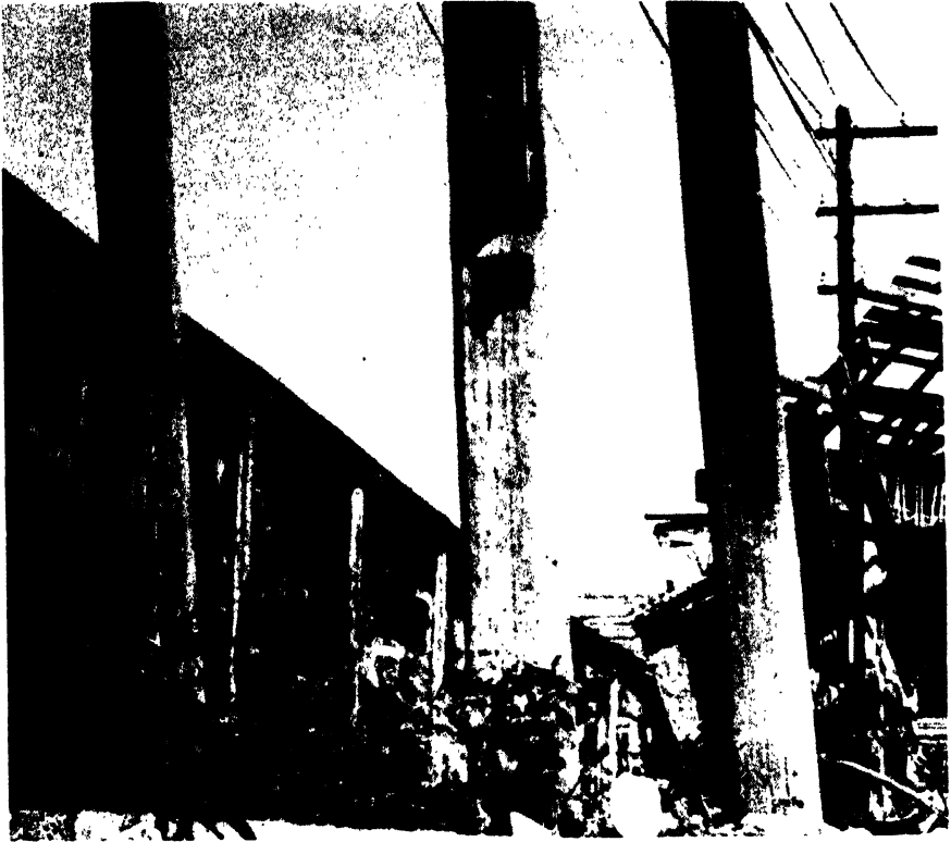
Figure 6.63b. Flash burns on wooden poles, 6,200 feet from ground zero. The uncharred portions were protected from thermal radiation by a fence.
