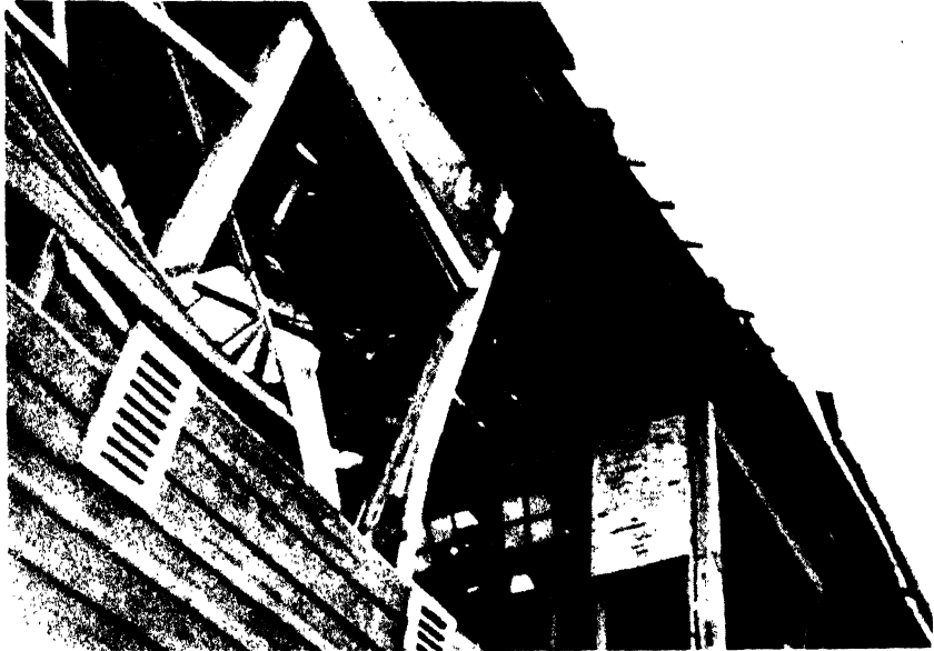
Figure 5.66a. Upper photo: Wood-frame building, 8,000 feet from ground zero, showing rupture of columns at points where windows or other horizontals were mortised in. Lower photo: Detail of above, showing typical column failure. (Note mortise and tenon joints at wall plate.)
