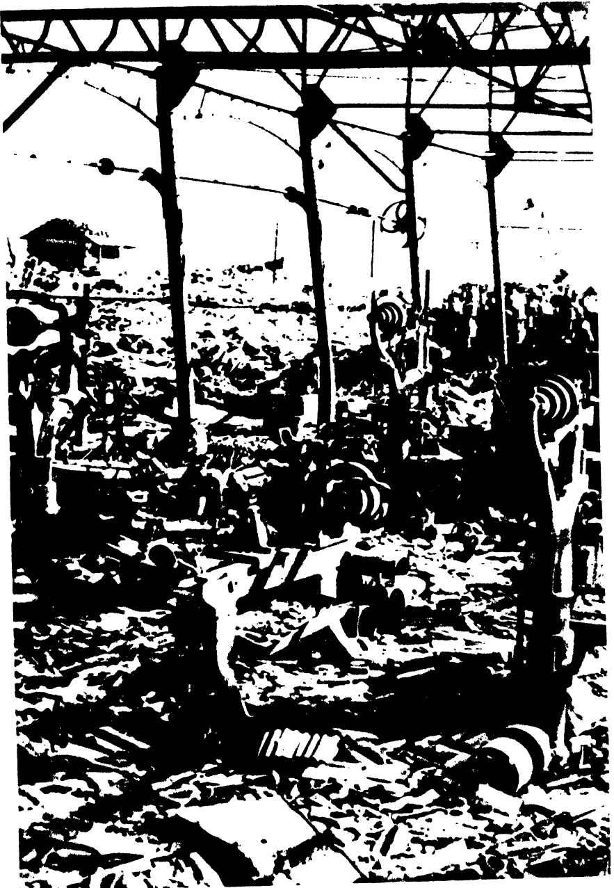
Figure 5.63. Steel-frame light engineering shop, 3,300 feet from ground zero. Machine tools rendered useless by fire, blast, and debris.
