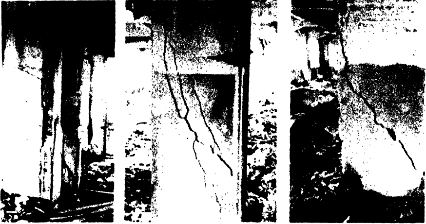
Figure 5.56d. Typical examples of column failure in reinforced-concrete frame building, 1,900 feet from ground zero.
