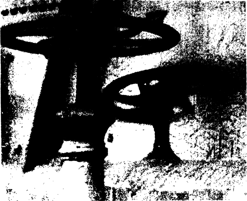
Figure 6.64b). Paint on gas holder, 7,000 feet from ground zero, scorched by the thermal radiation, except where protected by the valve.
