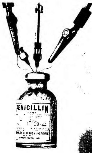
Fig. 38. Penicillin bottle used as titrating vessel. 4
