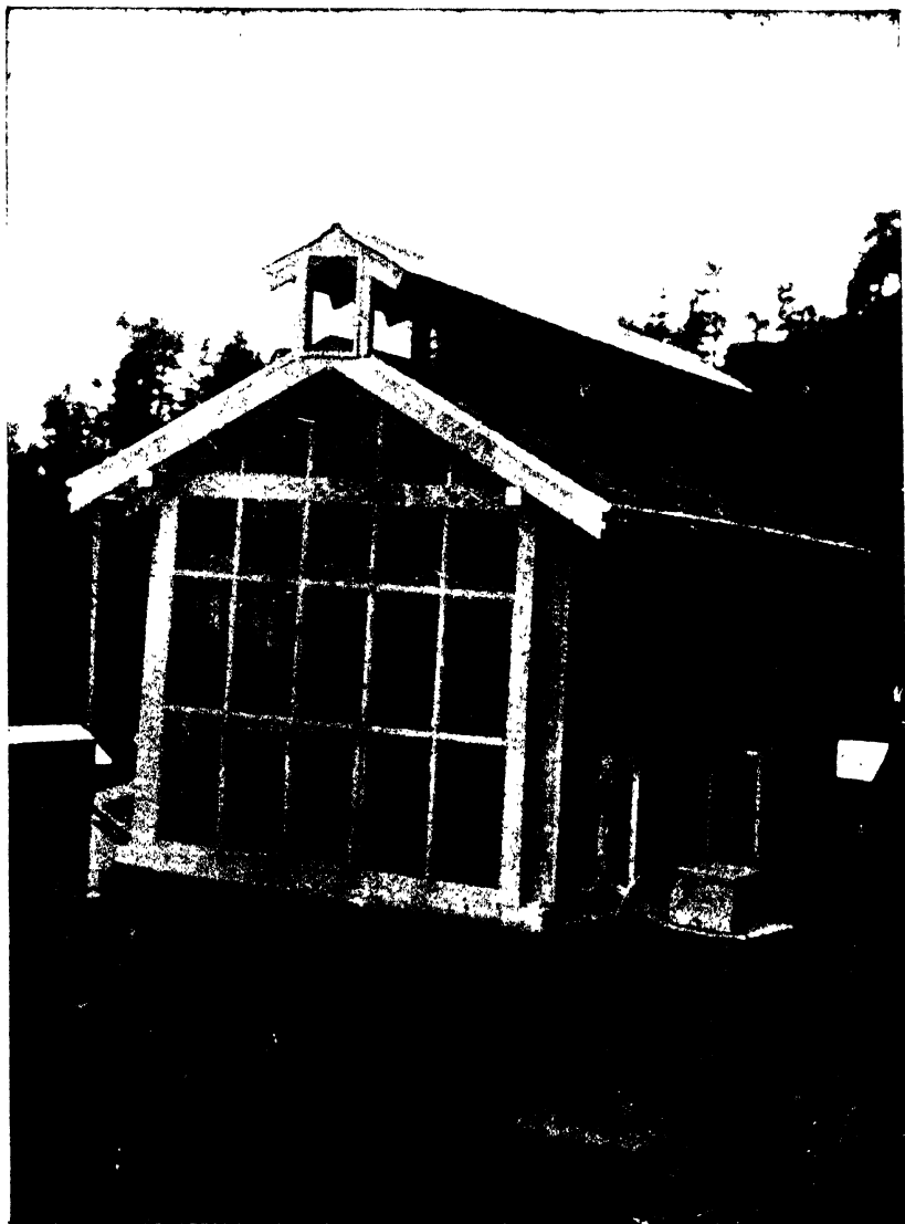
The cool green house at Simla showing double glass walls and roof with a space between the two walls. One of the khush boxes covered with muslin, the watering tank above it and three khush windows are also seen.
