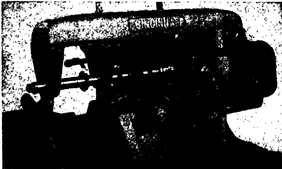
Fig. 96.—Fixture for roughing three gears at once.
