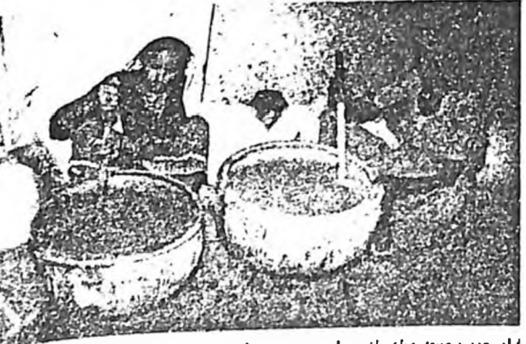
Natural stone colour being mixed with the two-year old processed lime in earthen pots. The churning continues for at least six months before application in the aaraish work.
