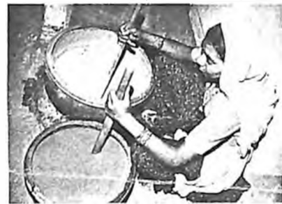
(From top) A lime jali being prepared; lime being ground with marble powder; and columns being made from crushed stones.
