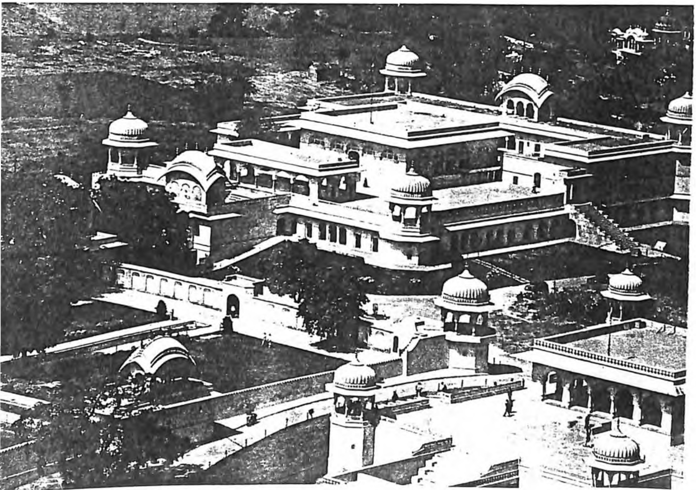
Govind Deoji Temple after restoration
