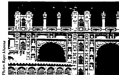
A recently constructed screen wall over the Zenana Kund at the Galta temple complex is laid with aaraish in relief work using different colours for motifs
