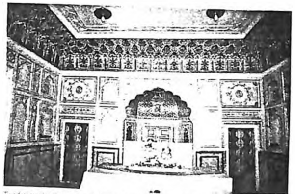
Traditional arts of decoration added to the interior of the garbha griha of Narayana Temple—in amalgam of mirror, silver, stucco, panni and meena work
