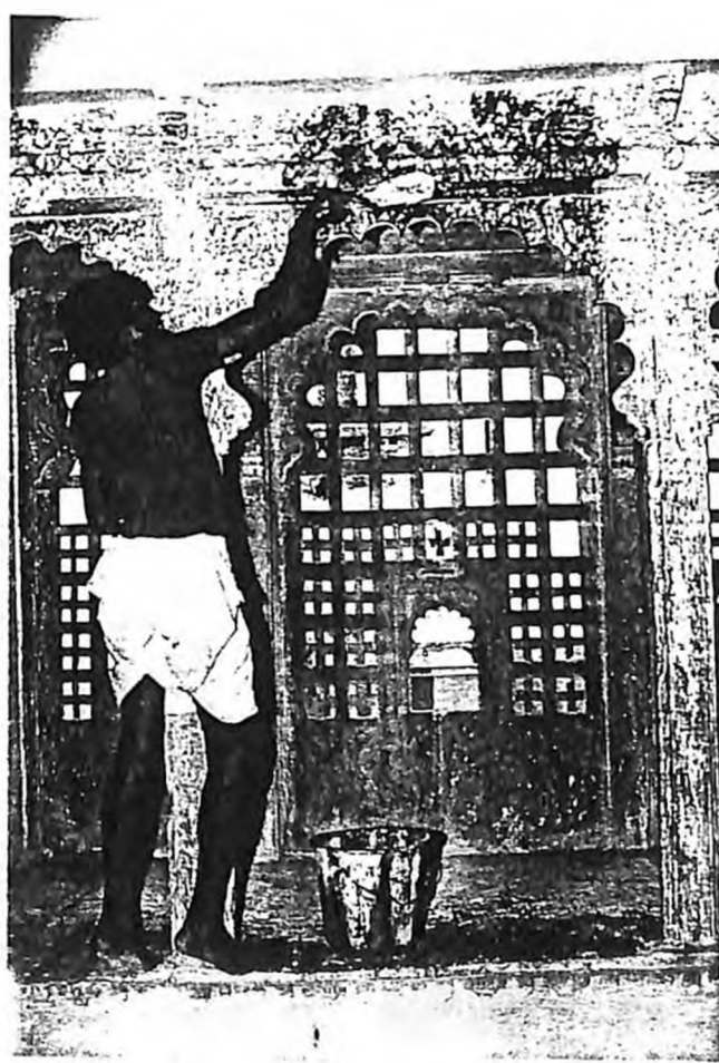
Left Temporary wooden supports were inserted where required. Below Cleaning the plaster off the stone walls. Below left Scaffolding over a jharokha prior to the application of lime plaster.
