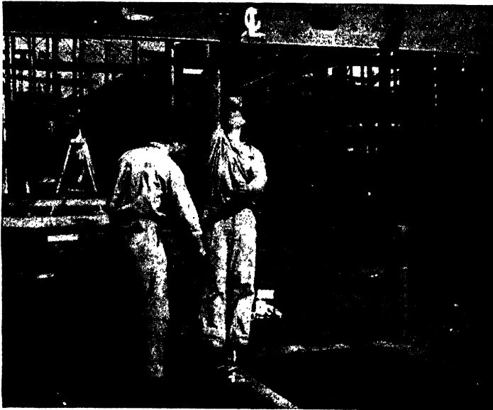
FIG. 351.—Setting transverse girder on center line.
