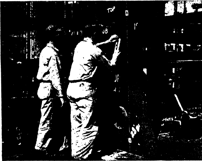
FIG. 348.—Web frame being set.
