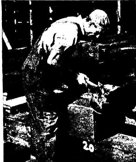
FIG. 284.—Keelblock toenailed preparatory to cutting to proper shape.
