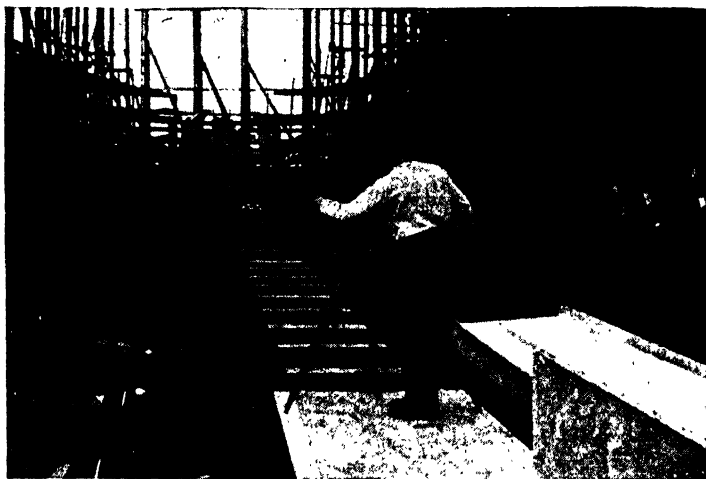
FIG. 286.—Establishing center line on keelblocks with engineer's transit.
