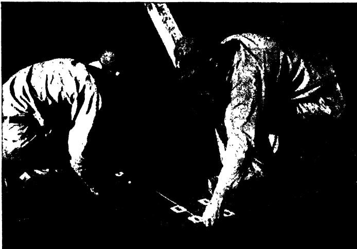
FIG. 315.—The shipwright establishing frame lines and 6-in. working line.
