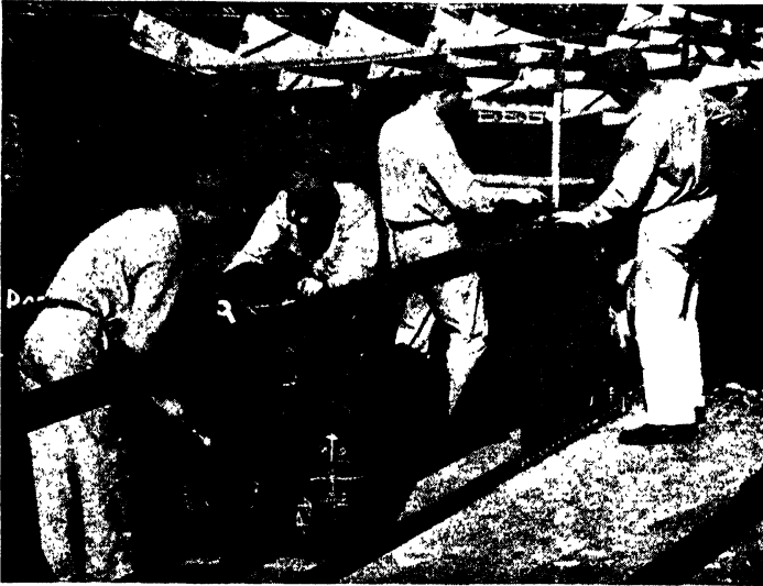
Fig. 326.—Shipfitters and shipwrights aligning and setting inner-bottom floors and longitudinals.
