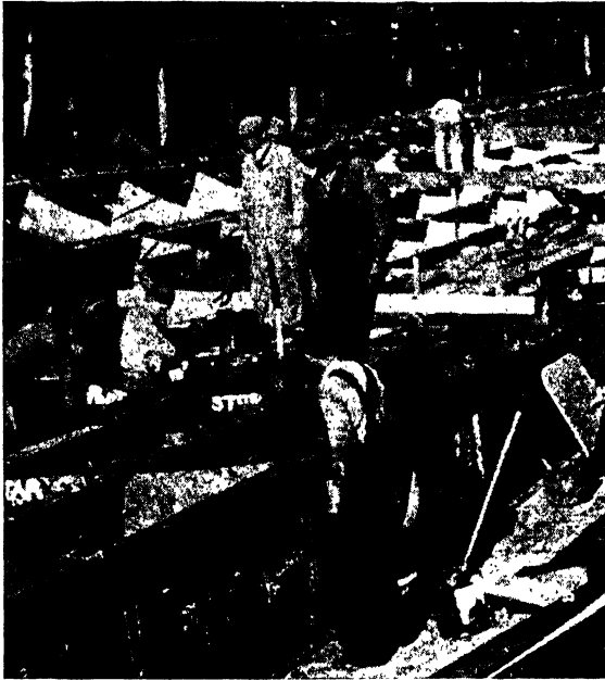
FIG. 328.—Shipwrights checking floors and longitudinals with height battens.
