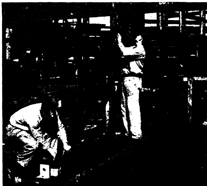
FIG. 353.—Shipwrights rechecking a transverse girder.
