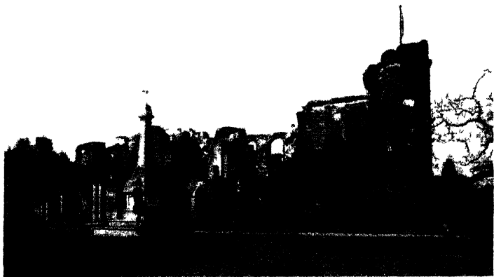
THE RESIDENCY, LUCKNOW
