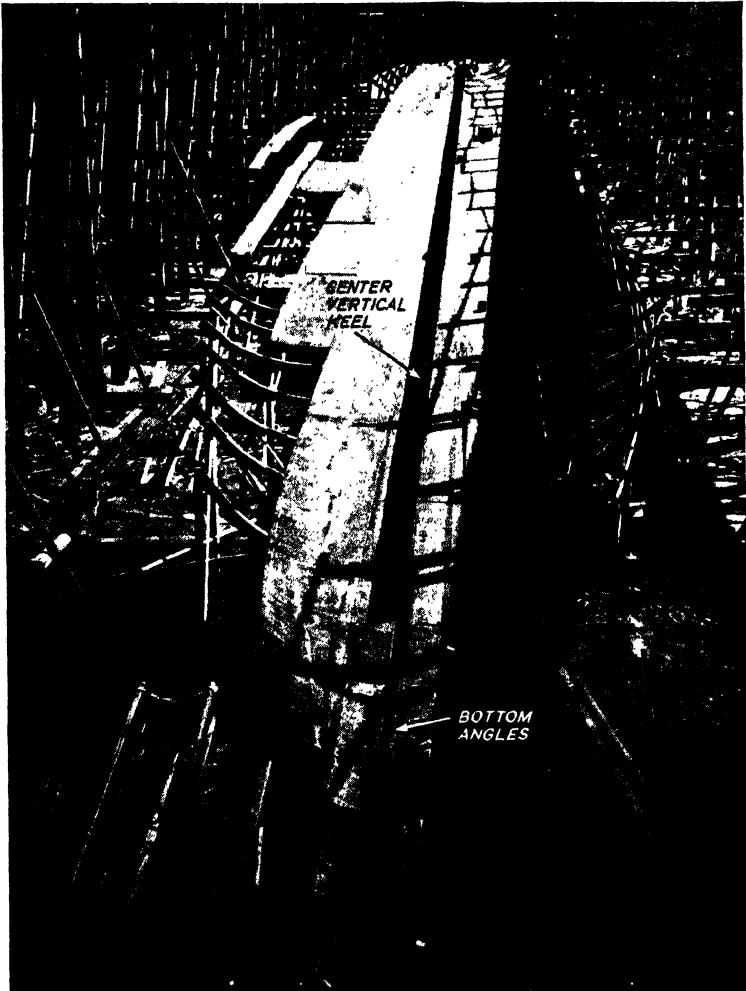
FIG. 54.—Center vertical keel. The flat plate keel has been laid and the center vertical keel is being fitted in place and attached by angle clips.
