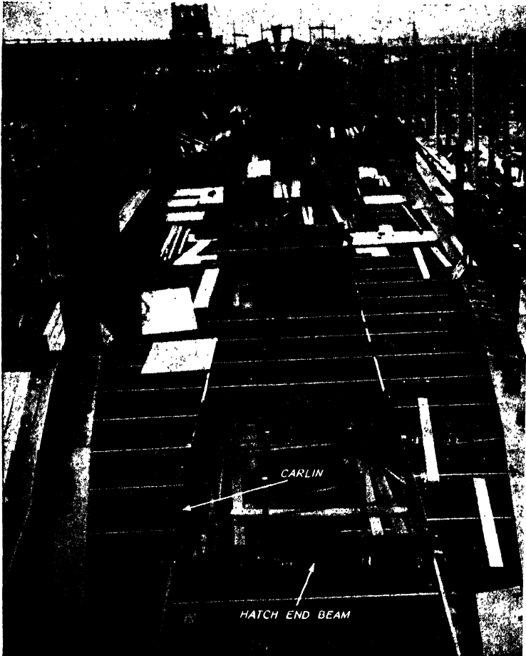
FIG. 80.—Deck beams. This is a photograph of the deck beams in place. Note how the beams are cut in way of the hatch.
