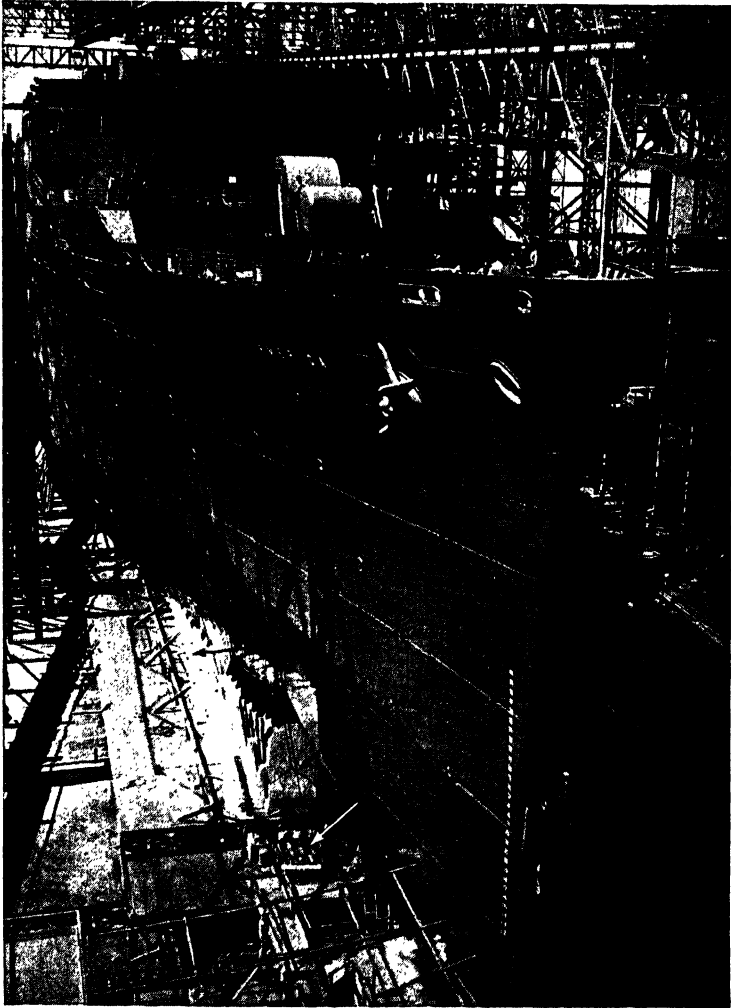
FIG. 162.—Bow view of vessel ready for launching. Note the relation between the size of the fore poppet and the vessel.
