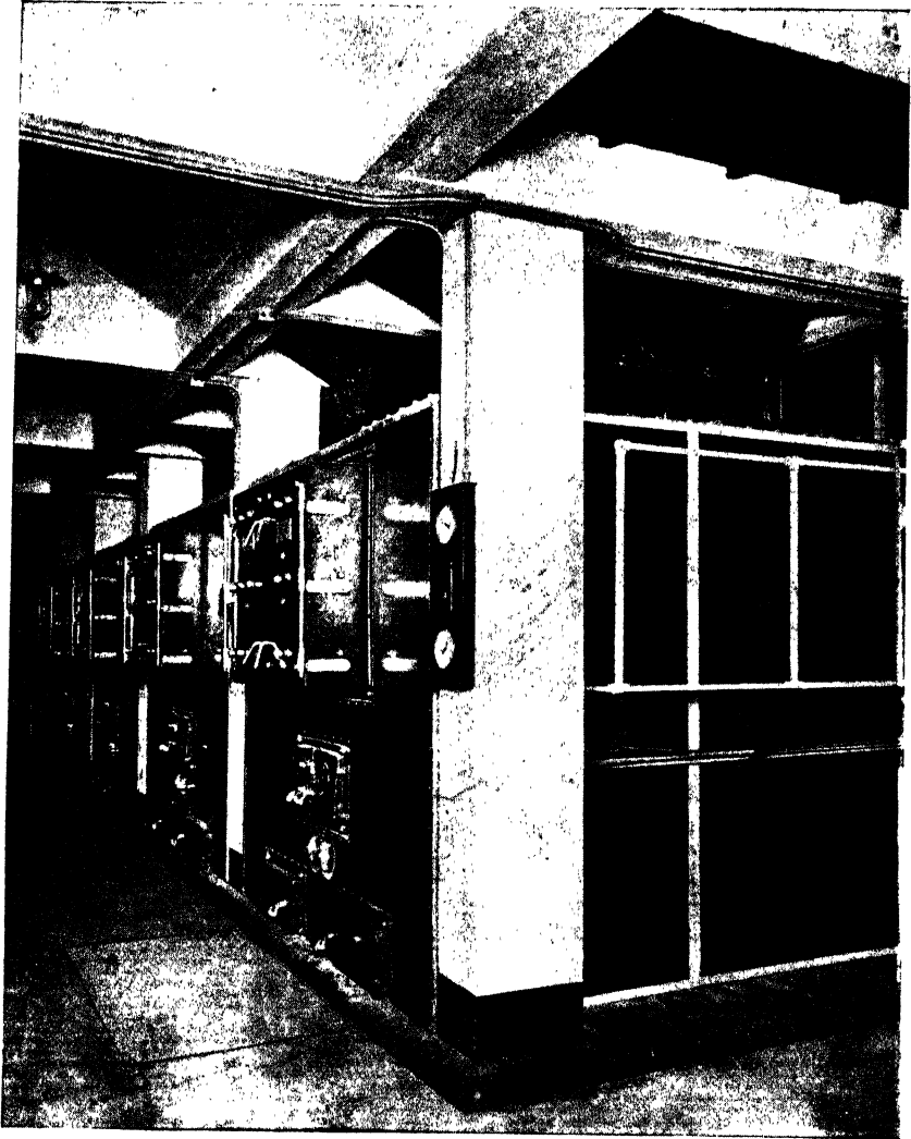
FIG. 33. A MAGAZINE TYPE BOILER INSTALLATION
