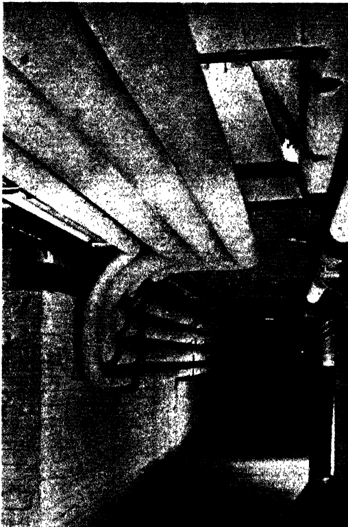
FIG. 91. PREFABRICATED PIPEWORK The change in direction of pipe runs is used for expansion purposes.
