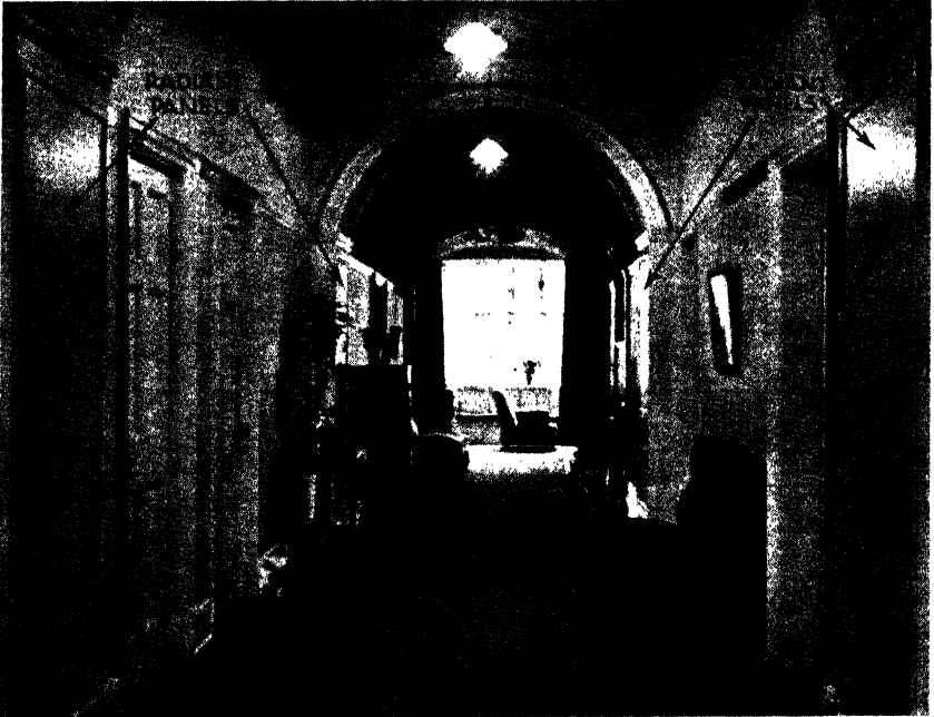
FIG. 18. CORRIDOR WARMED BY WALL PANELS OF THE SUPERIMPOSED TYPE
