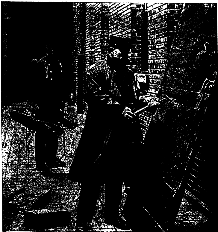
FIG. 5.—Fireman Cutting \frac{1}{4} -inch Steel Fire Door with Portable Apparatus.
