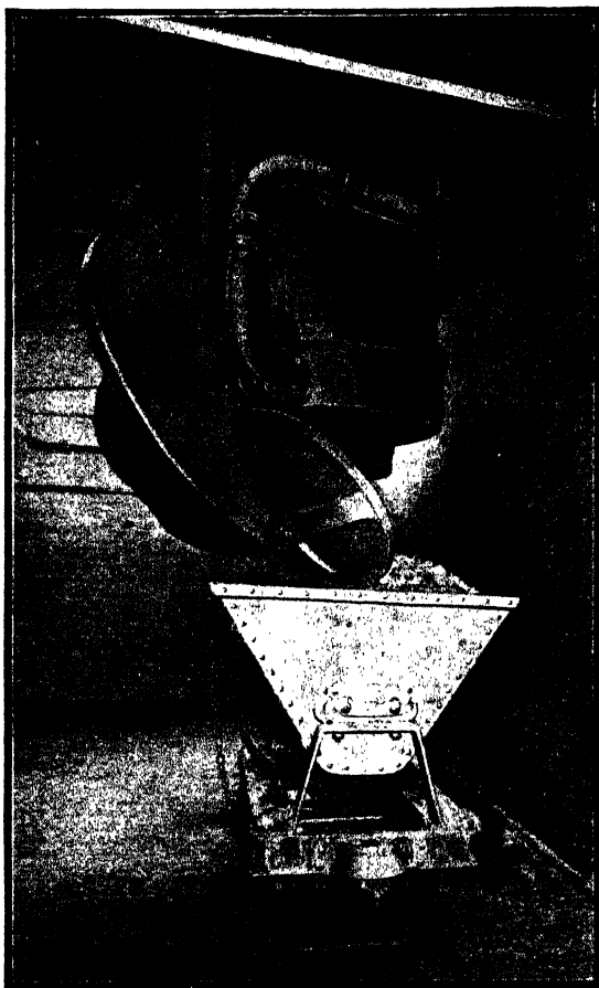
FIG. 7.—Beet diffusers (bottom part) showing doors and method of discharge of spent slices into lateral tilting trucks on rails en route for spent pulp silo (Fig. 10) (EGROT and GRANGÉ).
