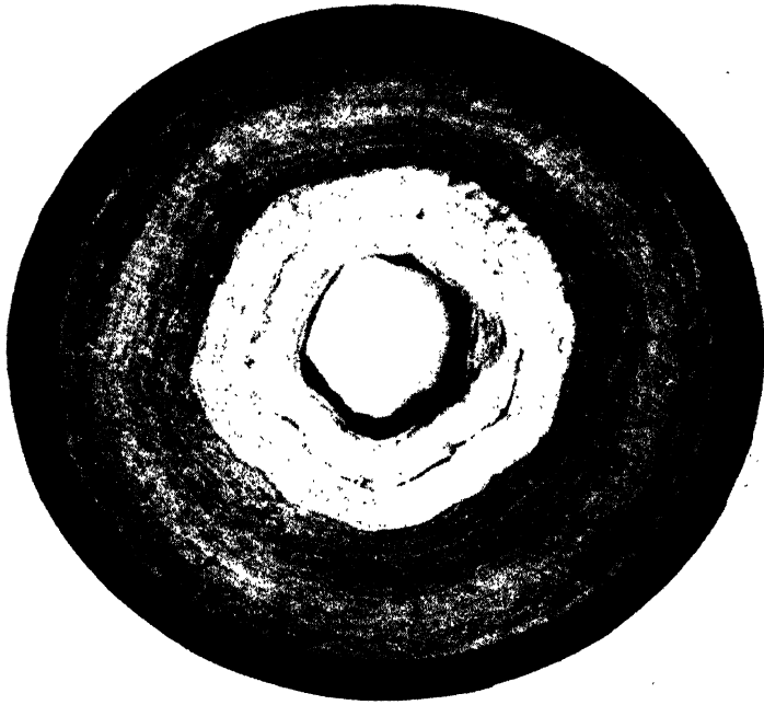
XI. HOT-WATER PIPE (3-INCH) NEARLY BLOCKED BY DEPOSITS OF CALCIUM CARBONATE (Repton, Derbyshire).
