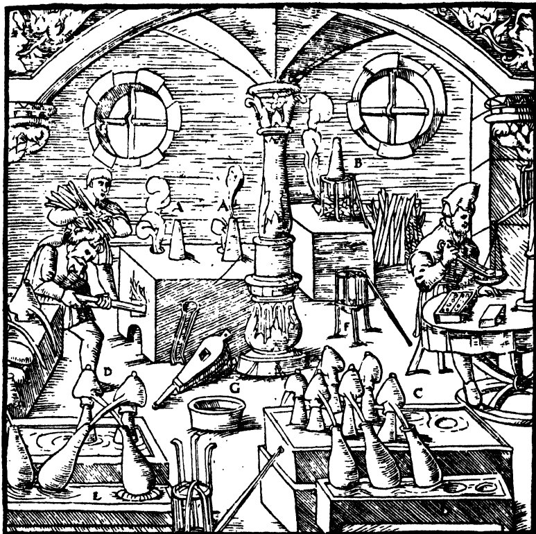
III A. MANUFACTURE OF ACID FOR THE REFINING OF GOLD. (Agricola: De Re Metallica , 1553.) The apparatus is not very different from that in use twelve centuries earlier and 200 years later.
