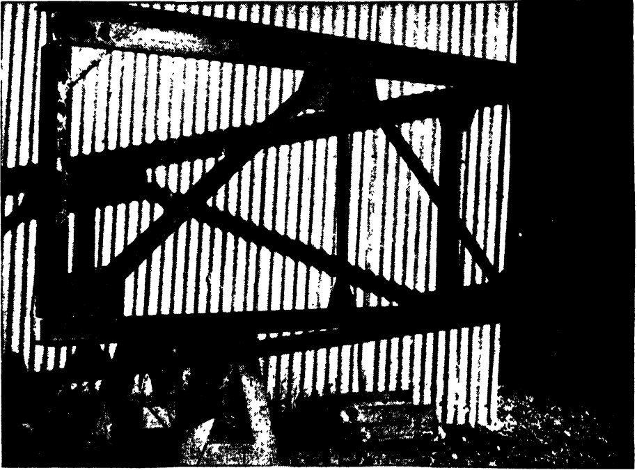
Figure 20-1 Riveted joints in steel construction.
