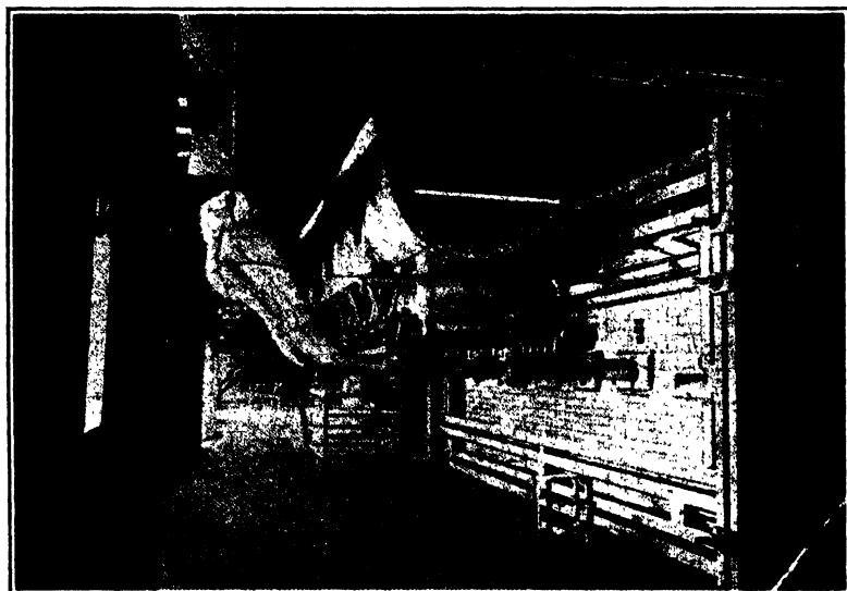
FIG. 142.—Firing end of Anaconda reverberatory furnace.
