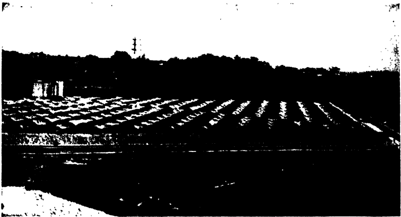
FIG. 187. A sewage-disposal bed in which the sewage is forced through sprays to hasten decomposition. Photograph by B. P. Domogalla.
