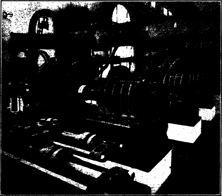
FIG. 100.—Multi-stage centrifugal boiler feed pumps. ( Platt Iron Works. )
