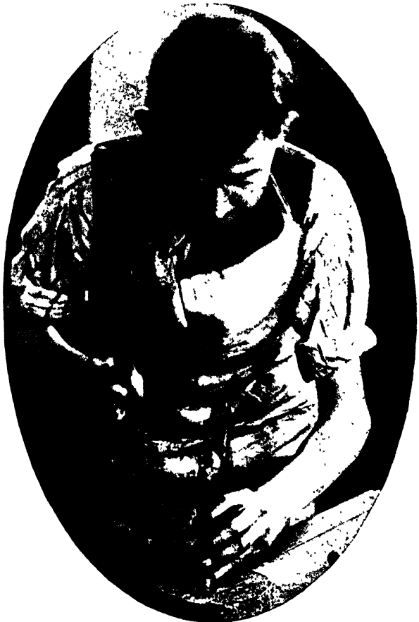
FIG. 51.—PUNCHING A HOLE IN TINPLATE ON A LEAD BLOCK.
