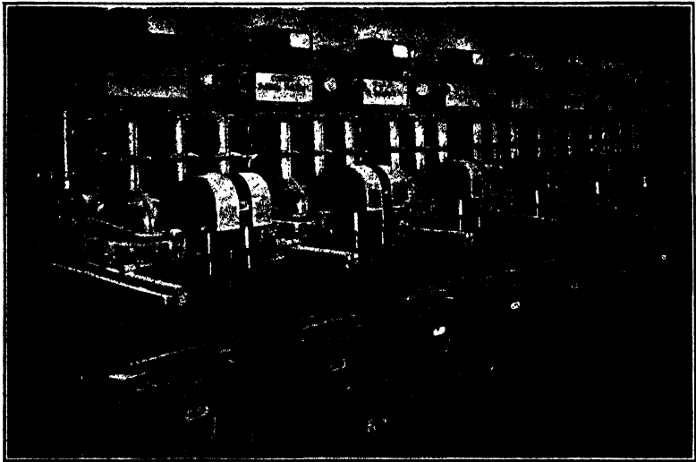
FIG. 200.—Installation of Reyrolle switchgear.
