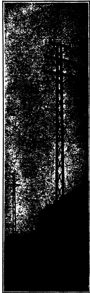
FIG. 273.—Steel-poleline. (Truscon Steel Company.)
