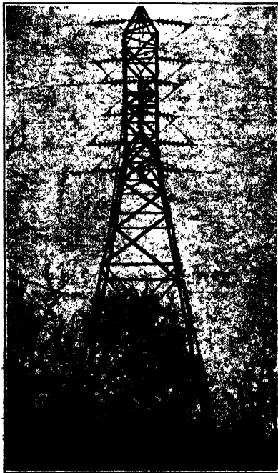
FIG. 289.—Transposition tower, Central Illinois Public Service Company. (Ohio Brass Company.)
