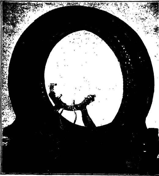
FIG. 45.—Stationary armature of engine-type alternator for diesel-engine drive. ( Westinghouse Electric Corporation. )
