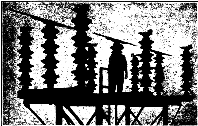
FIG. 348.—A 132-kv. 600-amp. motor-operated three-pole switch. ( Delta Star Electric Company. )
