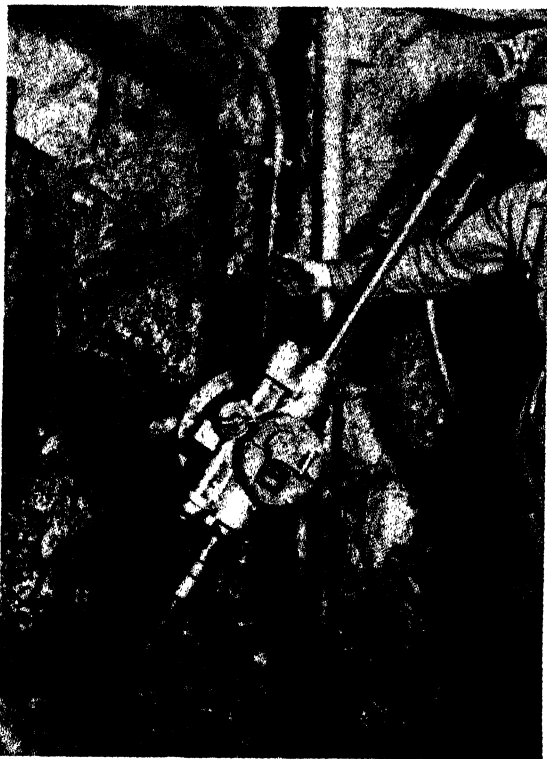
Fig. 14—Diamond drill operating underground. (Courtesy of E. J. Longyear Company)
