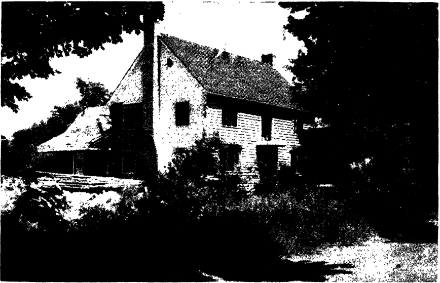
FIG. 2-13.—Remodeling a New England dwelling. ( Chase Brass & Copper Co. )
