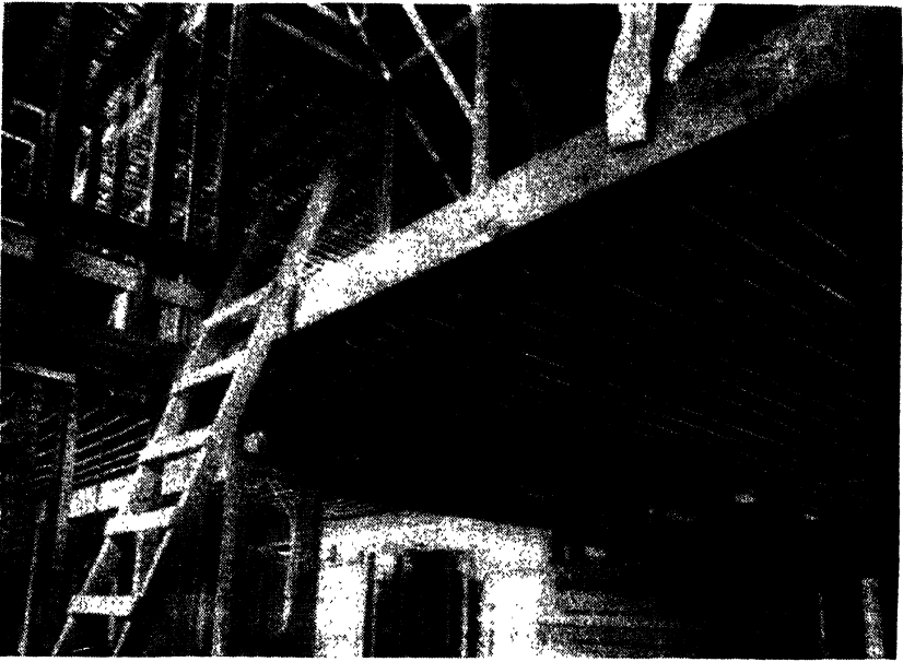
FIG. 2-14.—Installing copper coils in residence of Fig. 2-13. ( Chase Brass & Copper Co. )
