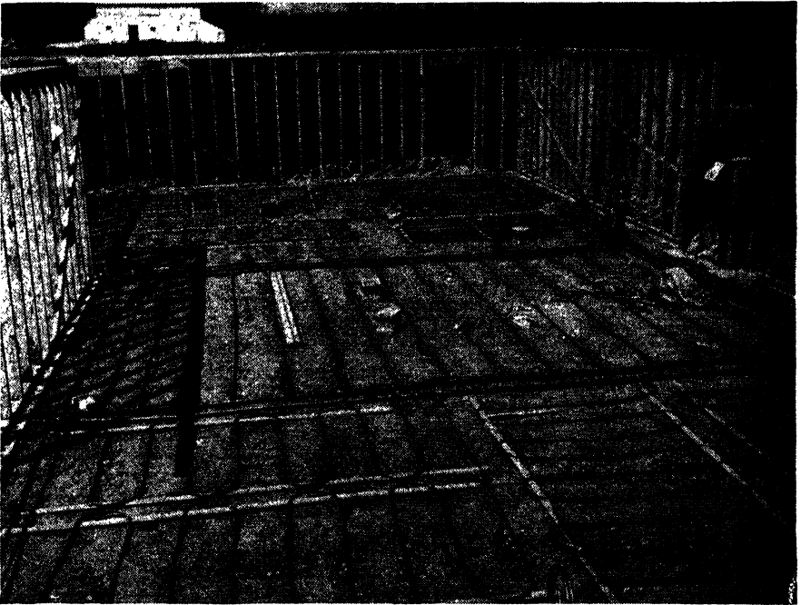
FIG. 4-4.—Combination grid and sinuous coils. ( A. M. Byers Company. )
