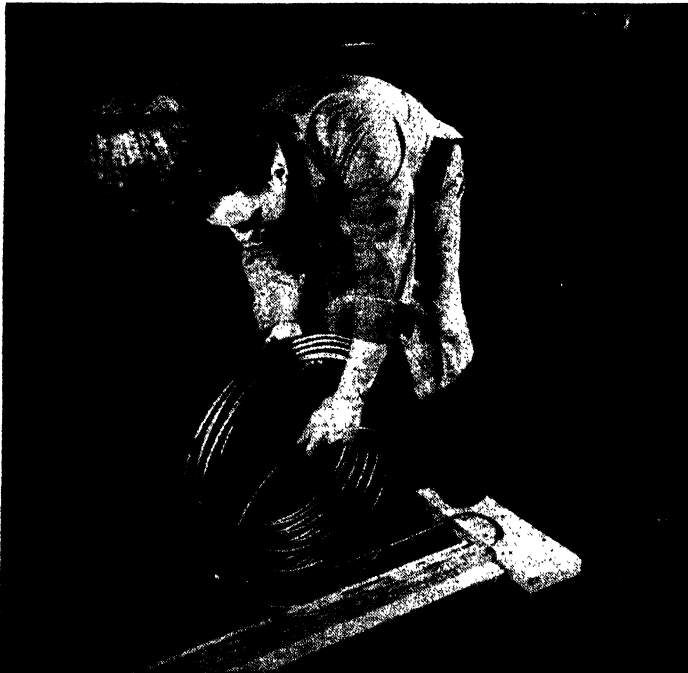
FIG. 8-25.—Forming copper-tube coils. ( Chase Brass & Copper Co., Inc. )
