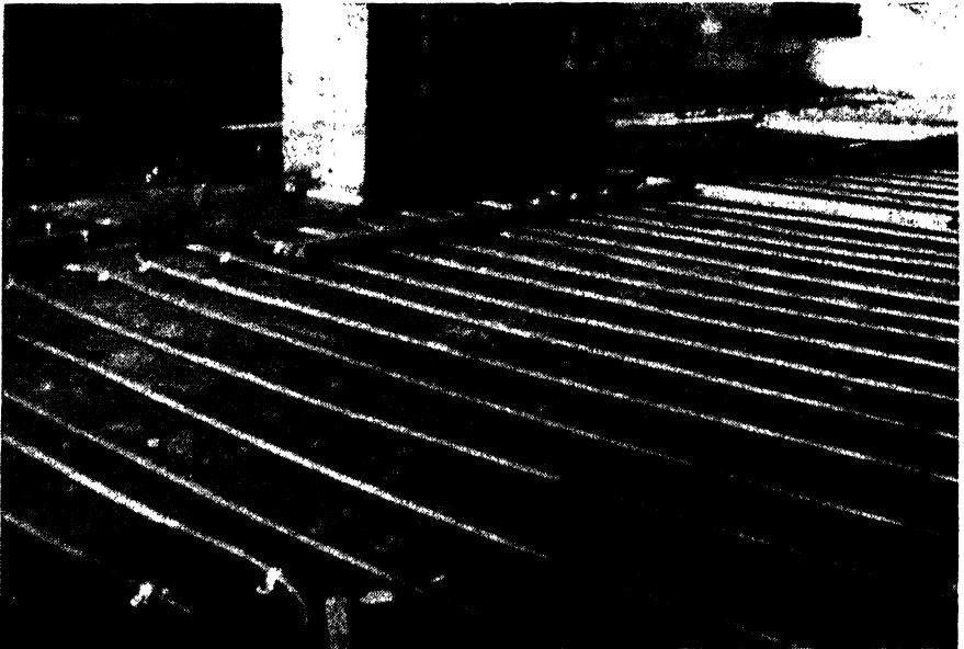
FIG. 8-12.—Coils laid on floor slab with insulation. (Chase Brass & Copper Co., Inc.)
