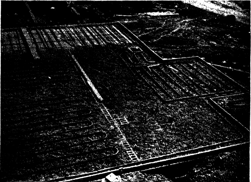
FIG. 4-5.—Wrought-iron floor installation. (A. M. Byers Company.)
