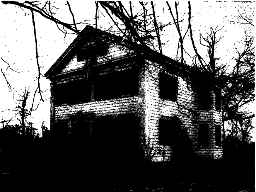
FIG. 2-15.—Radiantly heated pre-Revolutionary residence. ( Chase Brass & Copper Co. )
