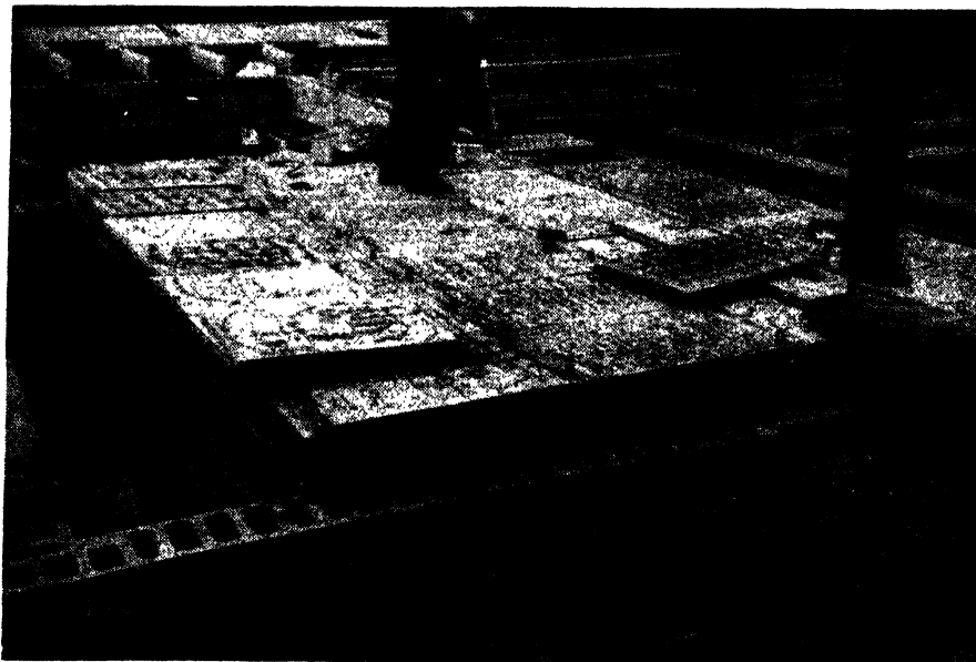
FIG. 8-34.—Prefabricated concrete-floor construction. (A. M. Byers Company.)
