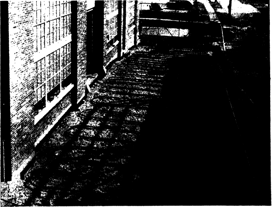
FIG. 8-38.—Snow-melting application in driveway. ( National Supply Company. )
