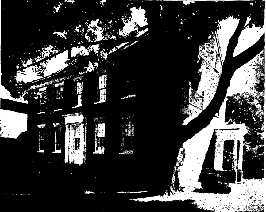
Fig. 2-17.—Pre-Revolutionary residence equipped with radiant heating. ( Chase Brass & Copper Co. )
