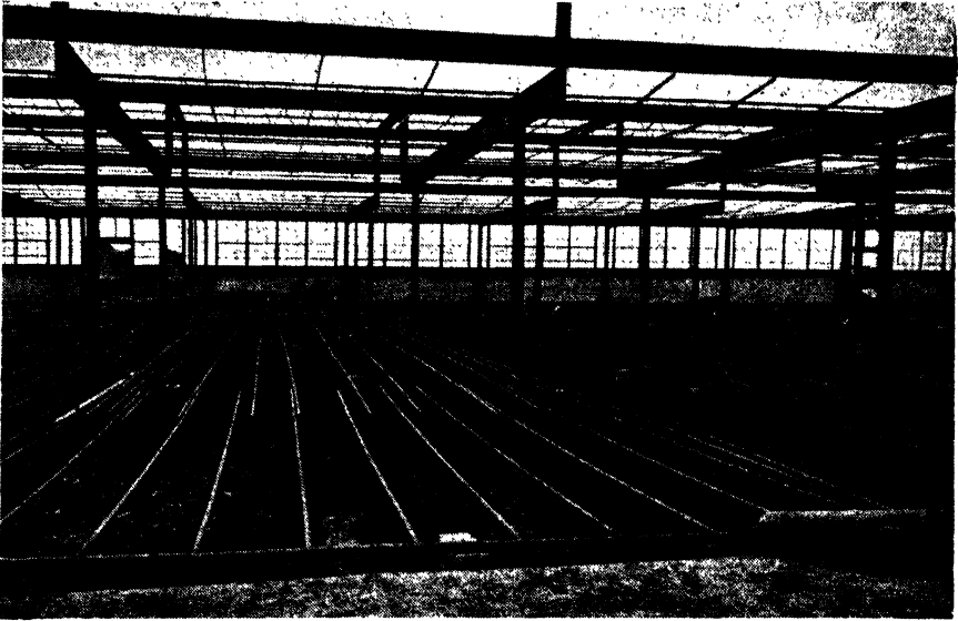
FIG. 8-31.—Installation of grid coils. ( A. O. Smith Corporation. )
