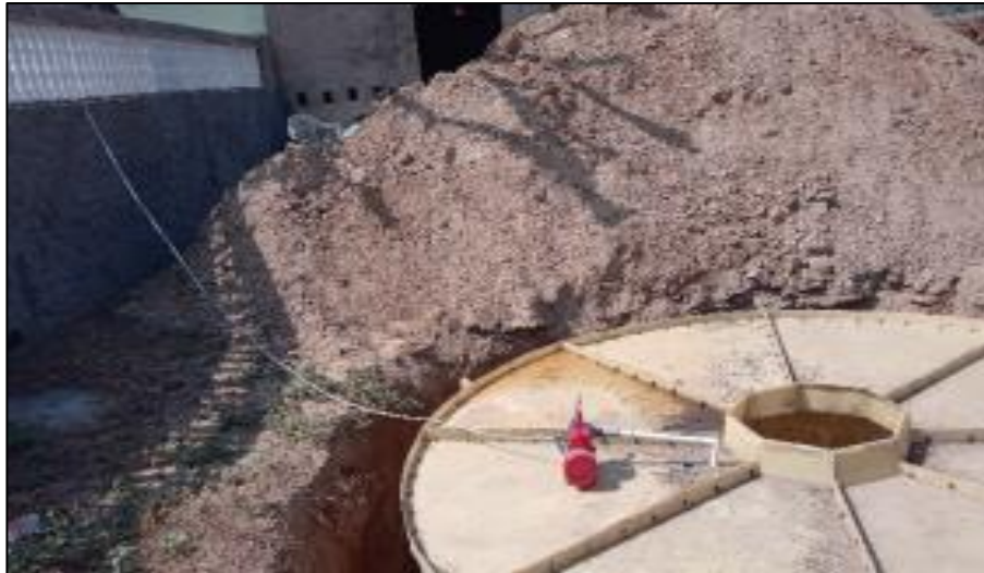
Figure 3-28 Fixing of a solar pump to the GFRP tank to draw water and ensure sustainable energy
