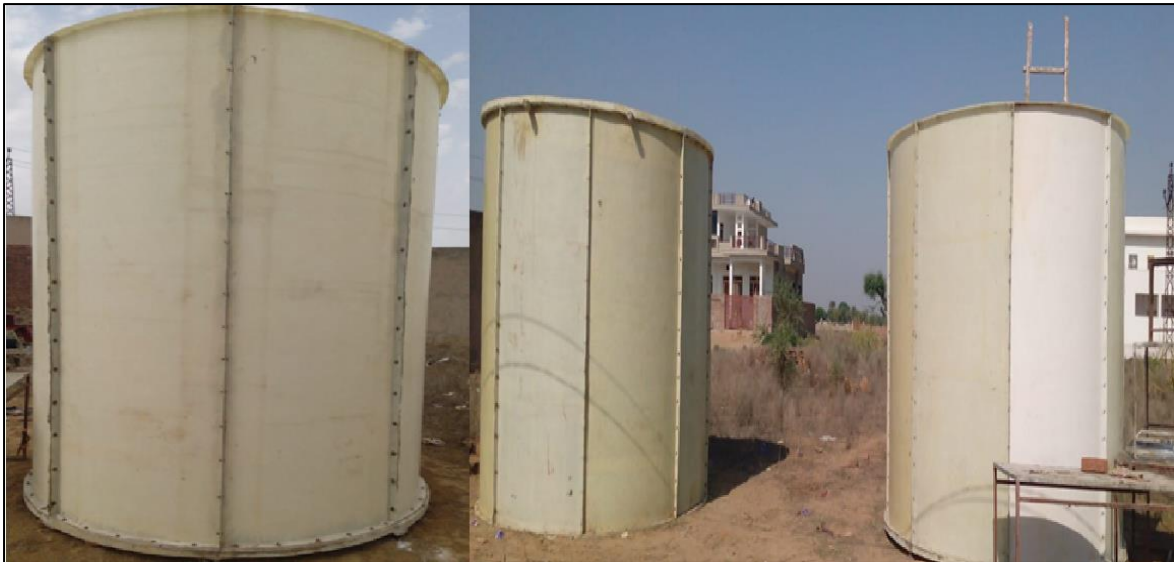
Figure 3-26 Assembly of GFRP tanks at the site of installation
