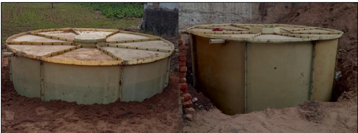
Figure 3-27 Installation of GFRP RWH tanks in a participatory household
