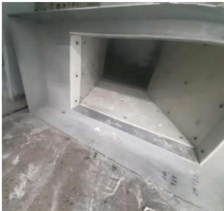
Fig. 6.11 Installation of UHMWPE liner sheets in the chute
