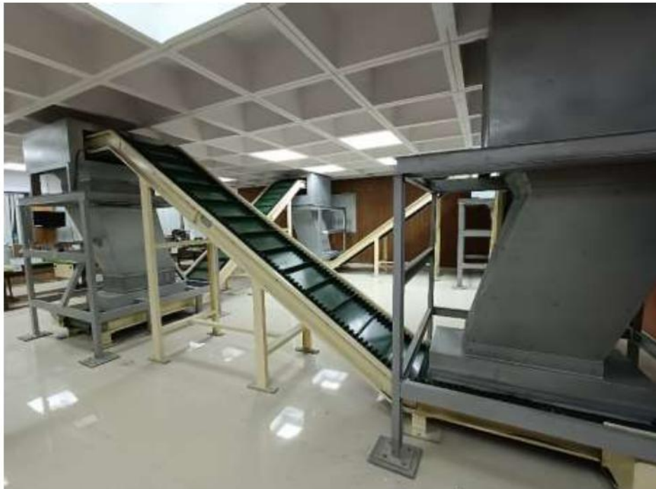
Fig. 6.16 Erection of complete system
