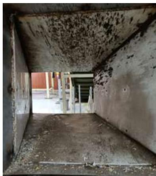
Fig. 7.10 Chute internal condition after running AFs at higher moisture
