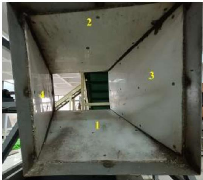
Fig. 7.17 Marking of liners in the flexible chute for wear measurement
