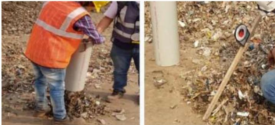
Fig. 5.4 Determination of angle of repose at site
