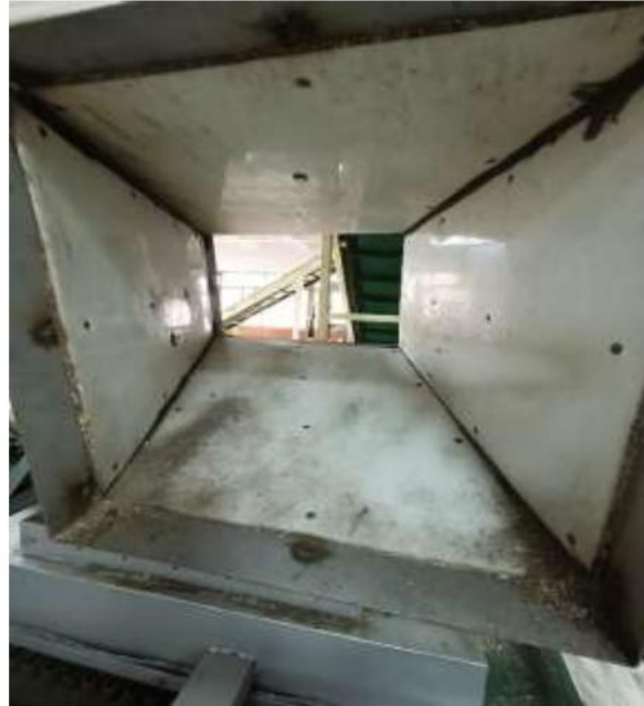
Fig. 7.6 Chute condition after an experiment for RDFs, industrial & agro waste at varying mass flow rates
