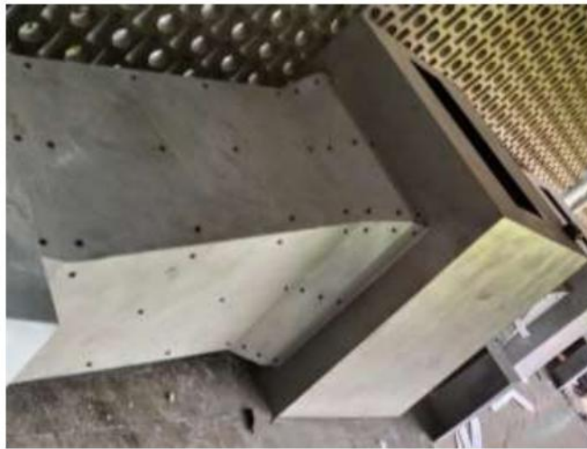
Fig. 6.12 Assembly of transfer chute
