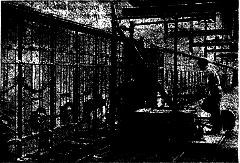
FIG. 13. Starch Kilns. (Courtesy Corn Industries Research Foundation)
