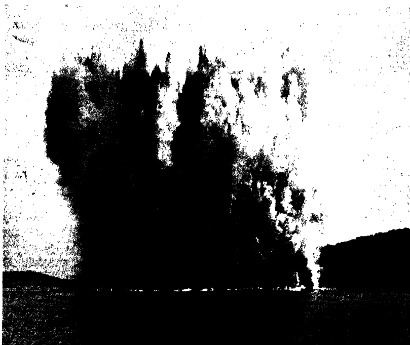
FIG. 3. Pipe Line Crossing Ditch Blast in Order to Lay Pipe Below Bed of River.
