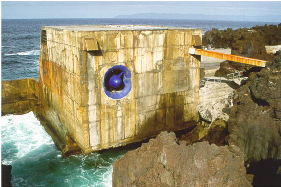
FIGURE 1.5: The OWC wave power pilot plant on the island of Pico, Azores, Portugal (Falcão et al. [3]).
