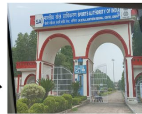
SAI North Regional Centre, Sonapat
