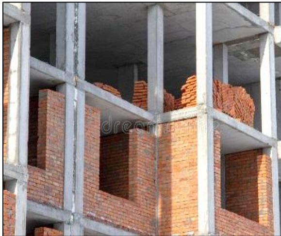
Figure 1.6. Masonry infill wall
