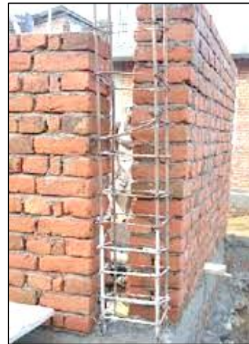
Figure 1.7. Confined masonry wall
