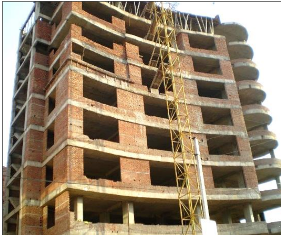
Figure 1.4. Construction of a typical MIW structure
