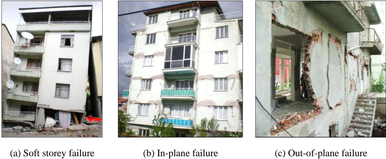
Figure 1.1. Adverse effects of earthquakes on masonry infilled RC buildings (Adem et. al., 2013)
