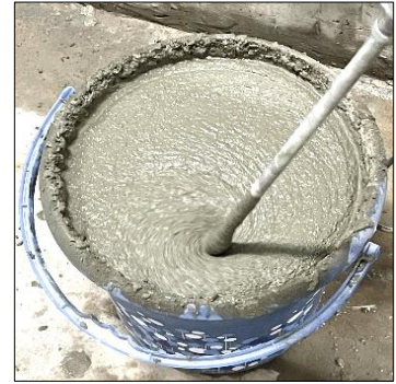
Figure 5.6(c) Mixing of plaster
