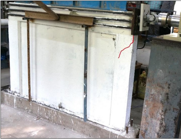
Figure 4.11(a) Diagonal tension cracks at the joint
