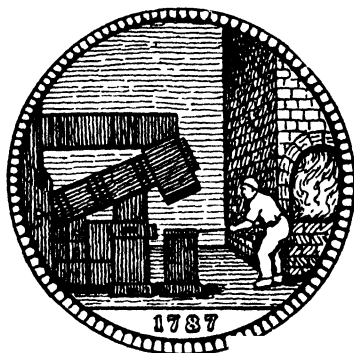
HAMMERING WROUGHT IRON
