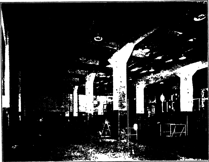
FIG. 194. Press Room, Chicago Daily News. Ceiling, including beams and ventilating ducts, finished in Johns-Manville "Sanacoustic Tile."
