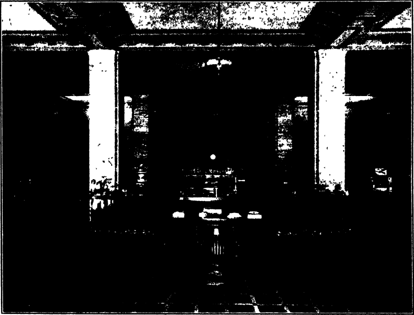
FIG. 198. Interior of Exhibition Room in Edison Building. "Kalite" plaster, 1\frac{1}{4} inches, applied directly to metal lath in ceiling.
