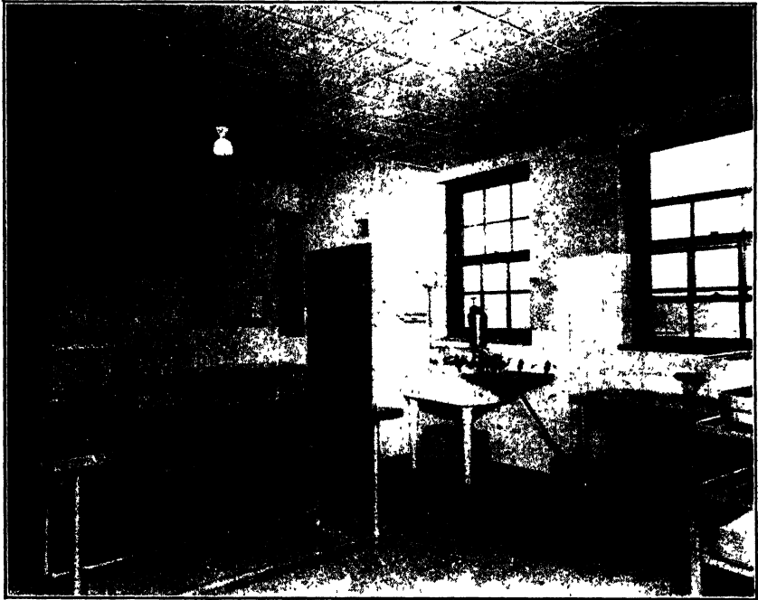
FIG. 201. Kitchen in Michael Reese Hospital. ( Schmidt, Garden and Erickson, Architects. ) Ceiling treated with painted "Acousti-Celotex."
