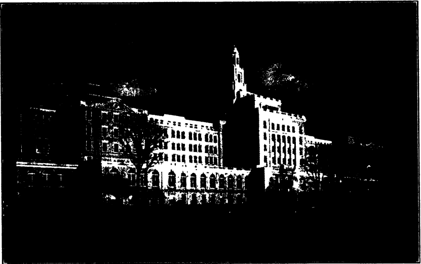
FIG. 199. Aetna Life Insurance Building. More than 300,000 square feet of "Acousti-Celotex," Type BB, used for acoustical treatment.
