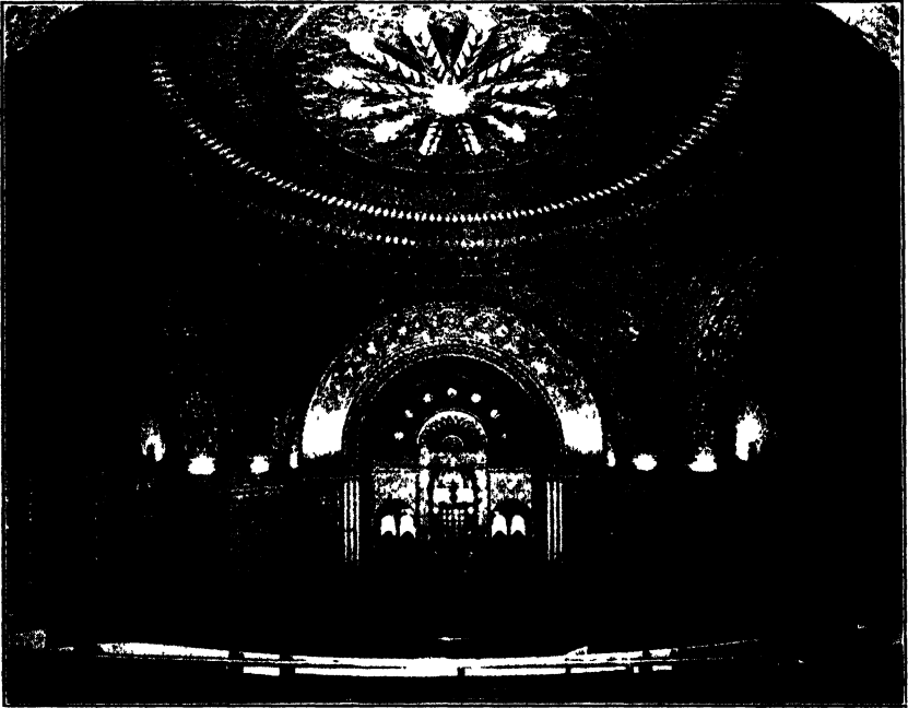
FIG. 213. Interior view of Rodeph Shalom Synagogue, Philadelphia. ( Simon and Simon, Architects. ) The entire ceiling above the spring line is treated with Johns-Manville "Nashkote," Type "C." White-faced "Akoustikos Felt" was used. The surface was sized and decorated.
