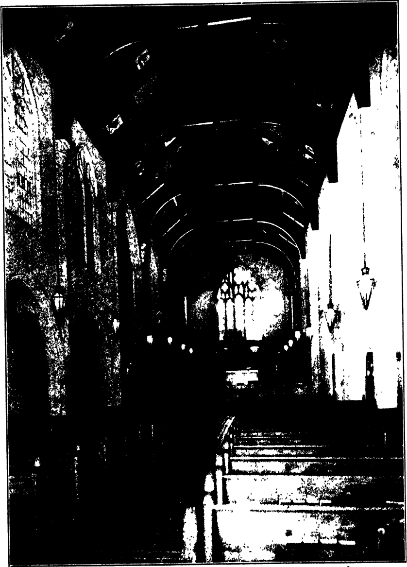
FIG. 204. St. Joseph's Episcopal Church, Detroit. Ceiling treated with Type B "Acousti-Celotex." ( Nettleton and Weaver, Architects. )
