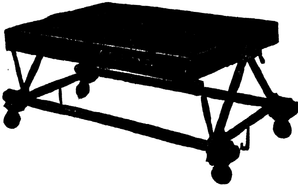
FIG. 1. Sun frame for blueprinting.
