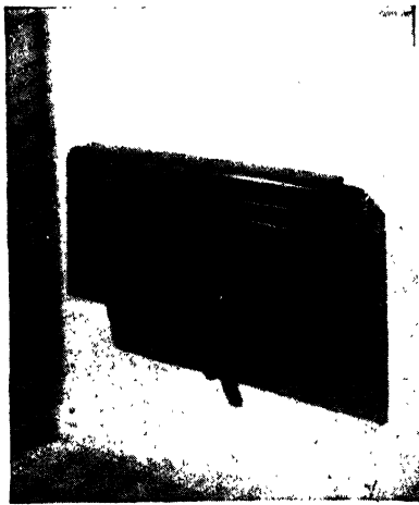
A neat background heater (flueless type) fitted in the hall.
