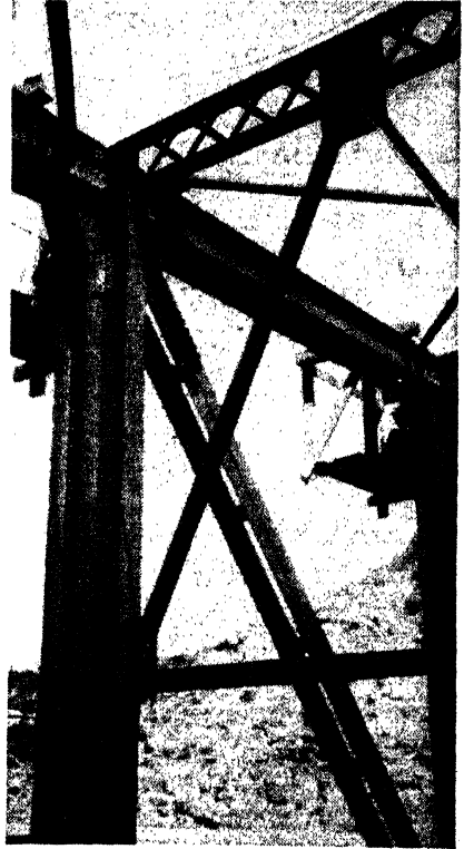
FIG. 16-25. Details of U5 of the north truss, showing the repairs made in another diagonal. Notice the single-angle lateral bracing, the heavy vertical members, and the narrow tie plates in the diagonal member. The wooden platforms are gage stations used for both mechanical- and electrical-gage work.
