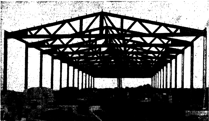
FIG. 9-16. Time-saving construction and low-cost erection were the results of a recently completed building of welded design to be used as a brass foundry by the Hays Manufacturing Co., Albion, Pennsylvania. Constructed of prefabricated trusses and columns, the building has a floor space of 11,645 sq. ft. and is 209 ft. in length and 52\frac{1}{2} ft. in width. The height from the floor to the bottom member of the truss is 17 ft.; and to the ridge of the roof, 34 ft. 7 in. (Courtesy of the Lincoln Electric Co., Cleveland, Ohio.)
