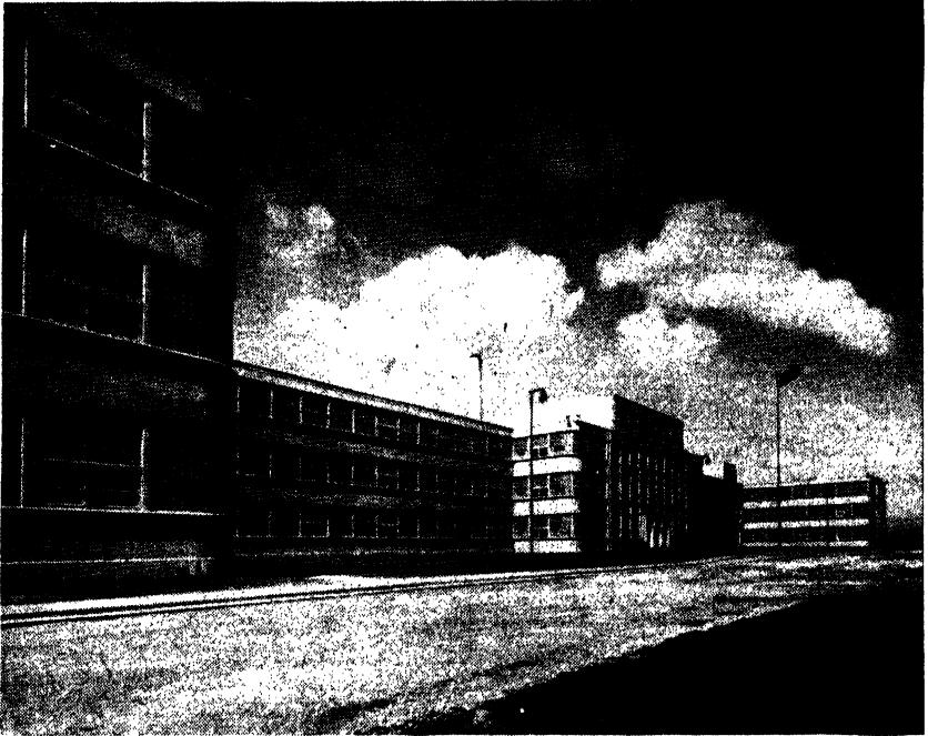
FIG. 5.16. Bell & Howell's attractive plant at Chicago, combining glass blocks for light and windows for ventilation. (Courtesy of Owens-Illinois.)
