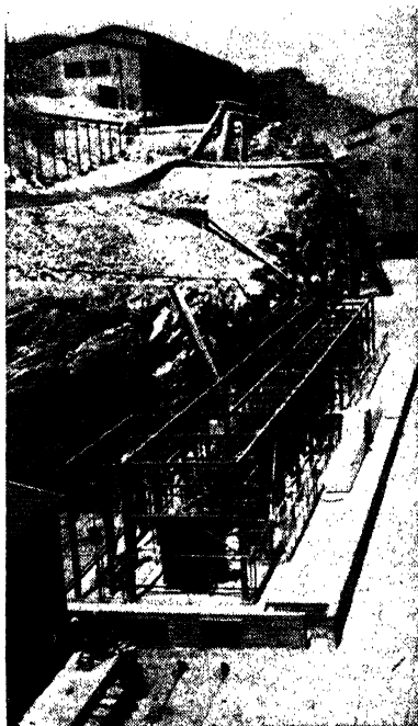
FIG. 4-8. Substation at the concentrator, Morenci Reduction Works. Notice the platform onto which the transformers may be skidded for handling by railroad.
