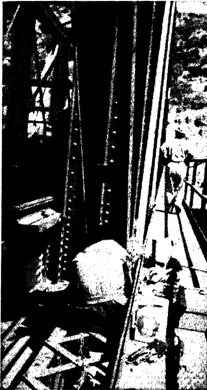
FIG. 16-19(a). Wiring some of the electric gages on the trolley beam near L7. The adhesive tape holding the wires is visible. The "live" rail is shown below the beam at the lower left.
