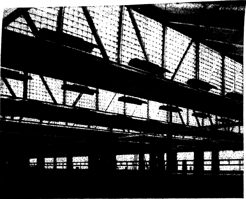
FIG. 5.13. This building has a saw-tooth roof with panels of glass blocks for daylighting and an excellent system of ducts for uniform ventilation of the extensive area. The bays are 25 ft. wide; the spacing of the duct openings 33 ft. This ventilation system is in the plant of the International Business Machines Corp. at Endicott, New York. It is the product of the Anemostat Corp. of America.
