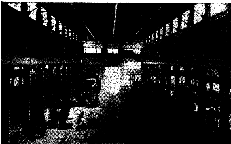
(b) View along the central aisle, showing the monitor and its windows. The light is coming in primarily from the right.
