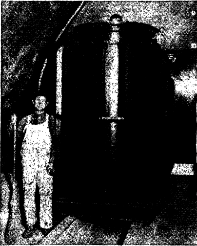
Fig. 4-9. A power transformer in the New Jersey ventilation building of the Lincoln Tunnel. (Courtesy of the Port of New York Authority.)
