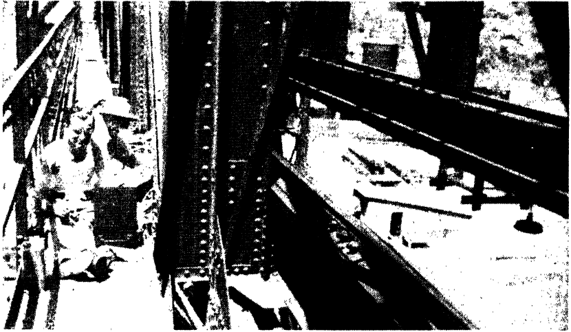
FIG. 16-6. Reading electric-wire strain gages at L7 of the south truss, where 12 separate gages were cemented to the trolley beam. The instrument with the handle contains the dials; the reading from each gage can be found by throwing a switch. Notice the details at the truss joint, and the north trolley beam in the background.
