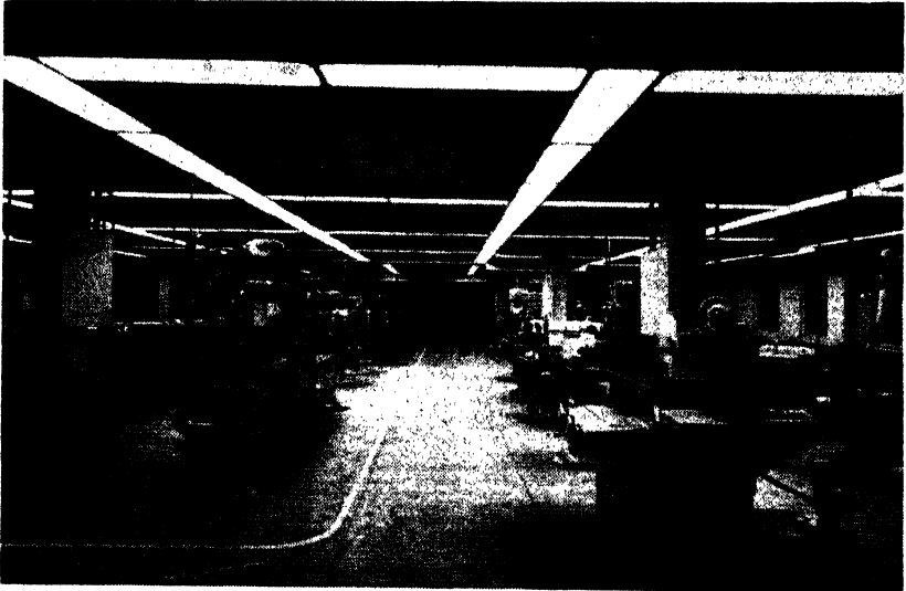
FIG. 4·22. This lighting system with its suspended-band arrangement provides excellent illumination at the machines. ( Courtesy of the General Electric Co. )
