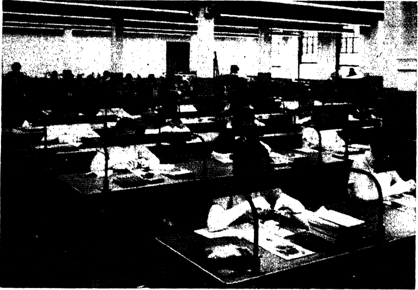
FIG. 4-4. An excellent illustration of supplementary lighting. There are fluorescent lamps in opaque reflectors below the eye level. (Courtesy of Matthew Luckiesh of the General Electric Co., and the Architectural Record.)
