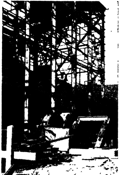
FIG. 9-7. Part of the secondary crushing plant of the Morenei Reduction Works. A 7-ft.-diameter Symons cone crusher is being lowered onto its reinforced-concrete foundation by the crane high up in the 70-ft. building. Notice the bracing, the girts, the frame, and part of the equipment for the tandem drive of a large conveyor. (Courtesy of the Phelps Dodge Corp.)
