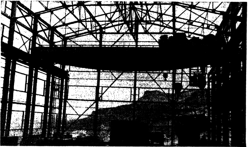
FIG. 9-35. A runway for a 150-ton crane, showing auxiliary columns under continuous crane girders. Notice the framing at the end of the building and the laced struts between columns at the lower chords of the roof trusses. (Courtesy of the Phelps Dodge Corp.)
