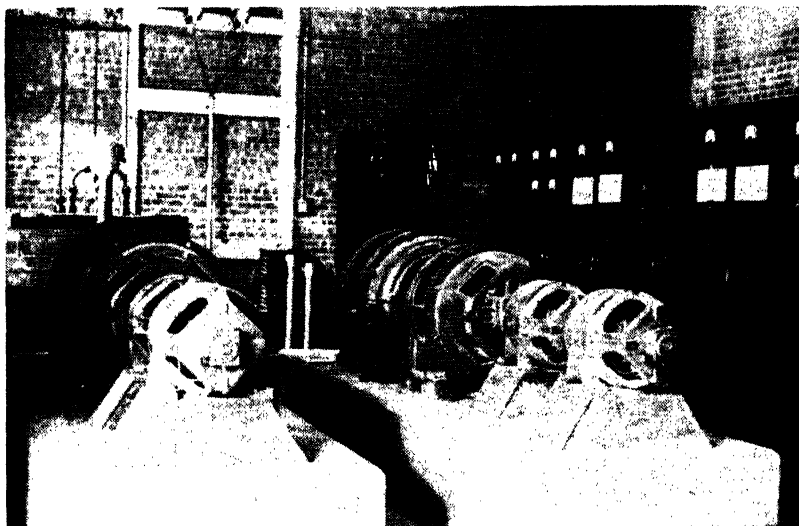
FIG. 4-10. Control panels and some of the electrical equipment in a control room. (Courtesy of the Phelps Dodge Corp.)
