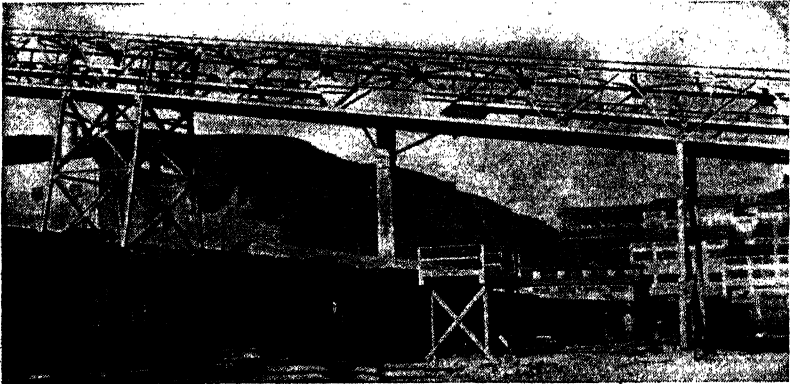
FIG. 15-16. Framing of a long conveyor gallery to the smelter at the Morenci Reduction Works. The anchor tower at the left is designed to resist all longitudinal forces; the other supports, like the one at the right, are to withstand vertical and transverse forces only. The central suspended chute is for loading cars if necessary. (Courtesy of the Phelps Dodge Corp.)
