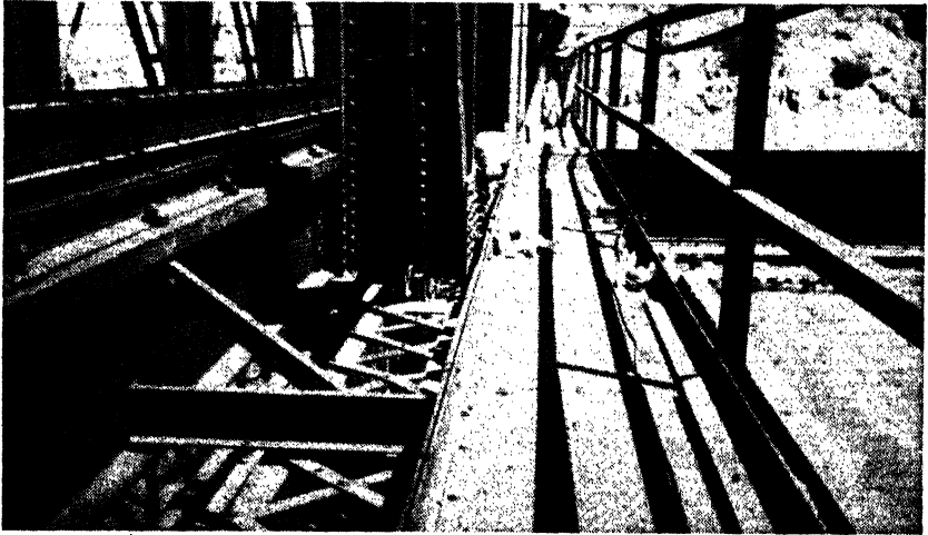
FIG. 16-18. View of typical trolley beam, intermediate bracket, chord, and sidewalk construction. Some of the lacing bars were bowed, but the cause of this is not certain.
