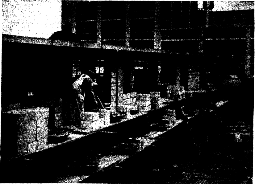
FIG. 11-28. Building a wall of high-pressure steam-cured cinder blocks with a cream-colored pigment, unpainted. The plant of the West Disinfectant Co. in the background is reinforced-concrete-skeleton construction with brick curtain walls. (Courtesy of Lone Star Cement Corp.)
