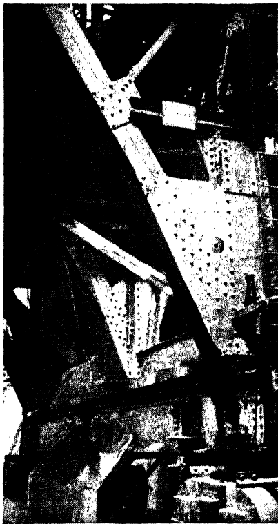
FIG. 16-11(a). Framing at the bottom of the tower. This view shows in the foreground the outer bent and the sliding bearing at the south end of the tower. The ore cars come next to the left-hand side of the tower.
