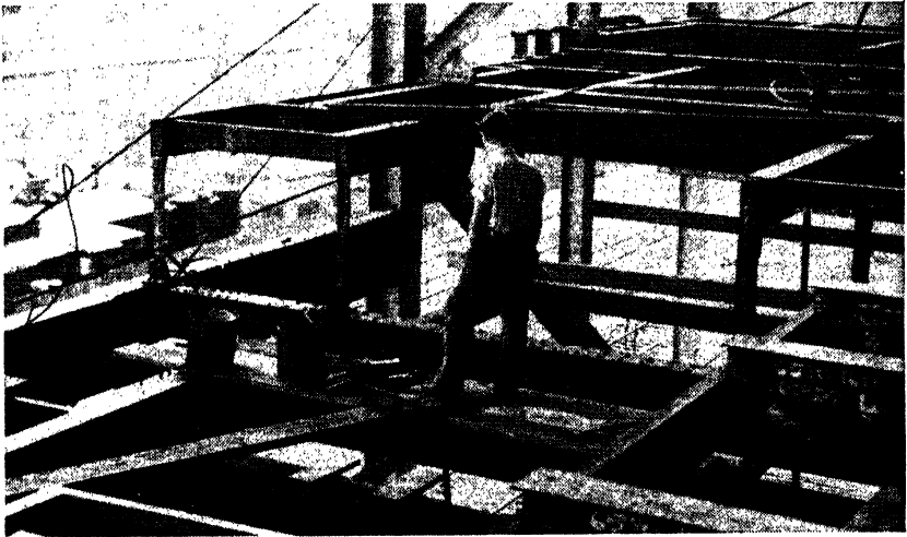
FIG. 10-8. Steelwork of the New Jersey ventilation building of the Lincoln Tunnel. (Courtesy of the Port of New York Authority.)
