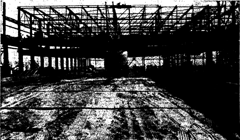
FIG. 9-1. Erection of the structural steel frame of a modern industrial plant having high-low-bay roof construction. One of the girders of the bridge crane is being raised. Notice the longitudinal bracing of the crane runway.
