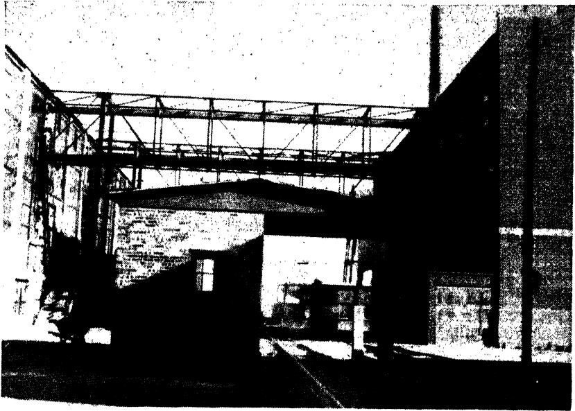
FIG. 4-19. A bus-bar bridge at the plant of the Phelps Dodge Refining Co., El Paso, Texas. A scale house is in the foreground.
