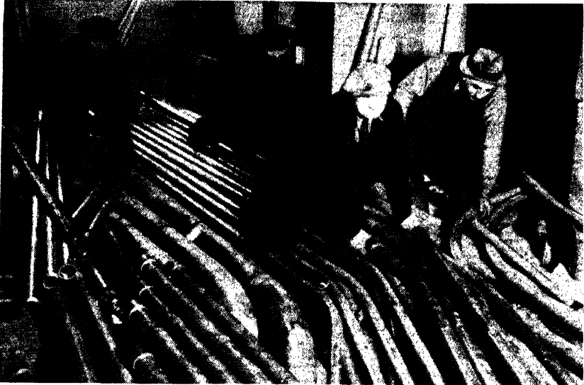
FIG. 4-16. Placing conduits from the control room to the pull chamber in the background for the future extension of the New Jersey ventilation building of the Lincoln Tunnel. (Courtesy of the Port of New York Authority.)
