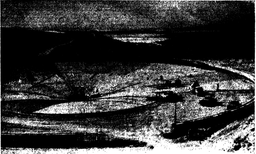
FIG. 11-25. The ring walls and bottom of a 300-ft. dewatering tank, showing the arrangement of joints. (Courtesy of the Phelps Dodge Corp.)
