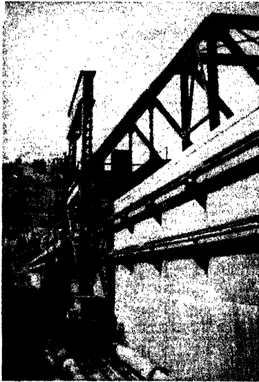
FIG. 16-23. The single-rail shear leg at the east end. The truss is hung from the top strut of the bent. The rods for measuring skewing forces connected the laced vertical posts to the bottom chords of the truss.
