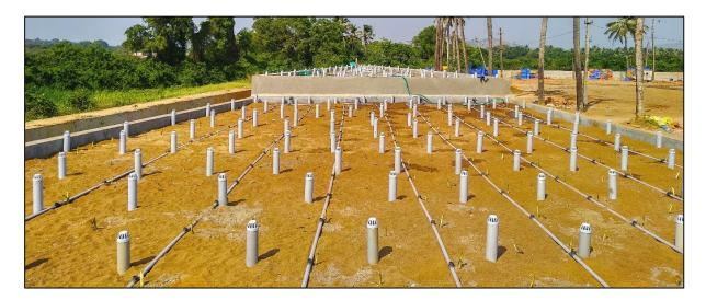
Fig 6.3: Two stage vertical flow wetland after construction
