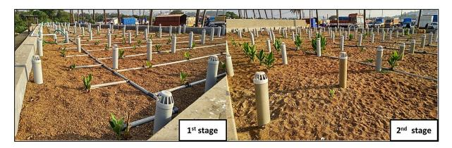
Fig 6.4: 1<sup>st</sup> stage and 2<sup>nd</sup> stage of vertical flow CW with *Canna indica* plantation
