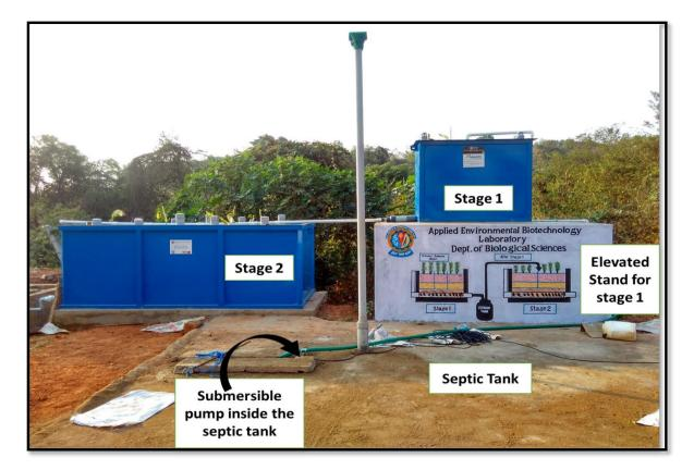
Fig 5.2: Design and construction of the wetland
