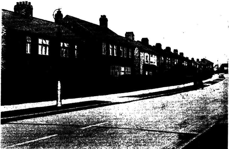
TWO TYPES OF HOUSES BUILT FOR SALE BY SPECULATIVE BUILDERS (Category 1)
