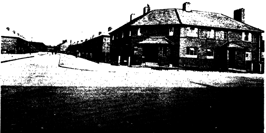
COUNCIL HOUSES BUILT ON THE SAME SITE (Occupied by tenants who previously lived in slum houses)
