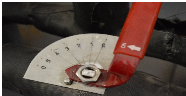
Fig. 4.6 By-pass valve to cater to the IHX
