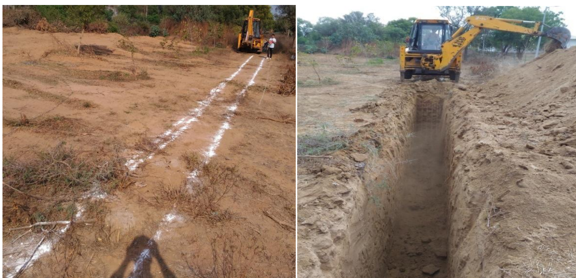
Fig. 4.11 Excavation work in progress and the trench excavated by excavation machine
