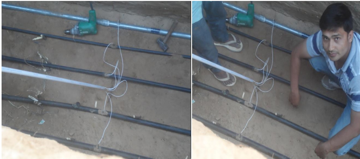
Fig. 4.13. Activity and position of RTD sensors placed along the length of EWHE pipes
