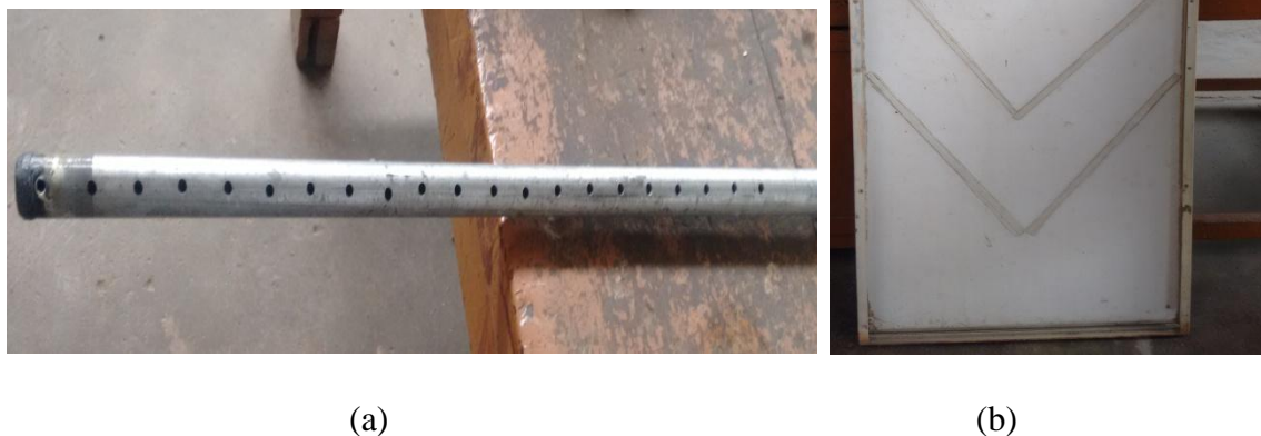
Fig. 4.6 (a and b). Fabrication of broad water channel collector (IPVTS)
