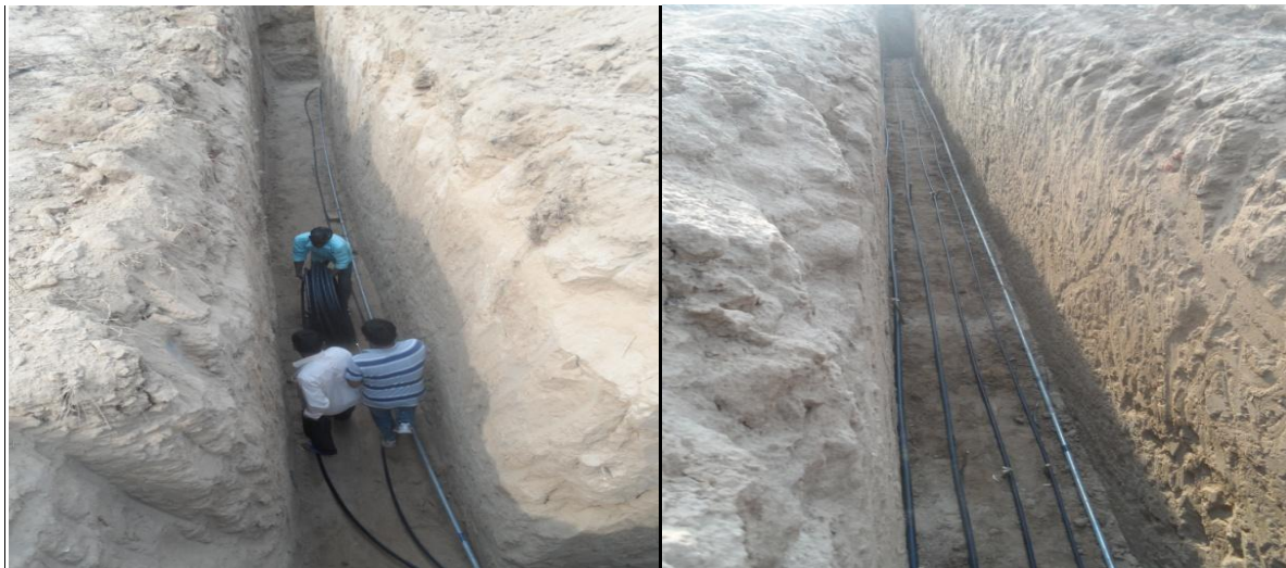
Fig. 4.12 Laying activity of EWHE pipes
