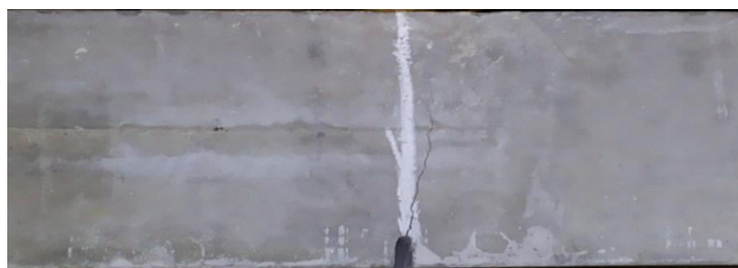
Figure 5.56 Crack propagation of SCC specimen with a/d ratio = 0.1
