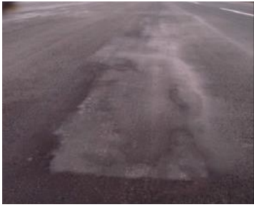
(a) Patching on runway
