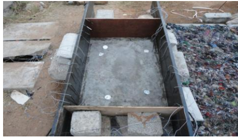
(i) Formwork layout for SCC with sensors
