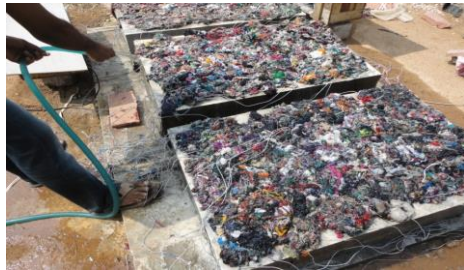
(iii) Curing of SCC Slab
