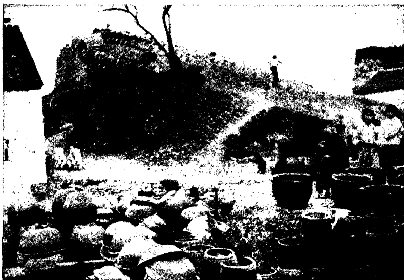
FIG. 123. A Chinese kiln with a number of sections. It is lighted at the bottom, the waste gases preheating the higher chambers, and the cooling of the lower chambers preheating the combustion air. The fuel is small chips of dry wood fed through the holes in the crown. ( Henry Jewett Greene. )
