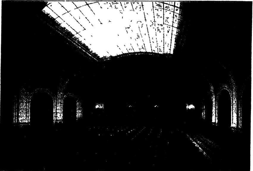
FIG. 8.37 — Arc Lamps above a Glass Ceiling
