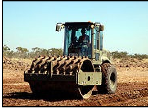
Roller Compactor at road formation
