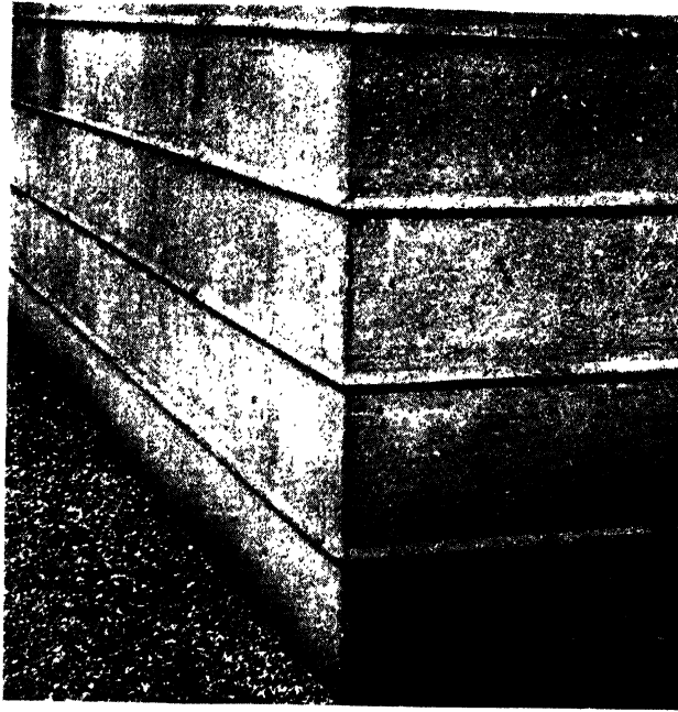
FIG. 173.—MARLBOROUGH COLLEGE: CONCRETE SHOWING MARKS OF WOODEN SHUTTER BOARDS AND CONSTRUCTION JOINTS HIDDEN BY VEE-SHAPED PROJECTIONS.
