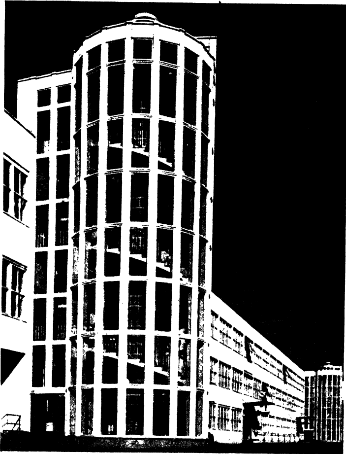
FIG. 6.—FACTORY AT STOCKHOLM, SWEDEN.
