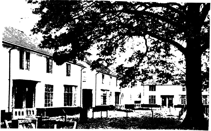
FIG. 21.— HOUSES AT WELWYN GARDEN CI
