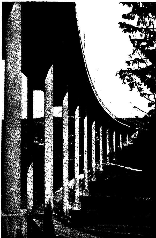
FIG. 13.—AN APPROACH TO SANDÖ BRIDGE.
