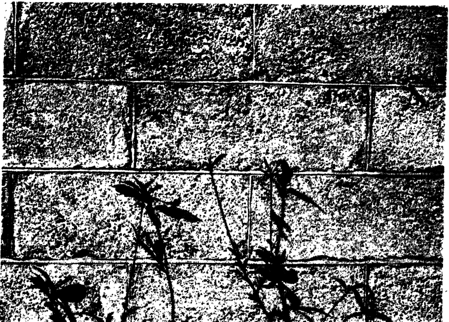
FIG. 164.—DETAIL OF A HOUSE IN DEVONSHIRE THIRTY YEARS OLD : THE SCRUBBED SURFACE HAS WEATHERED UNIFORMLY.
