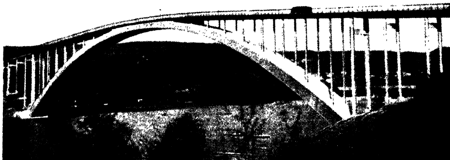
FIG. 12.—SANDÖ BRIDGE, SWEDEN.
