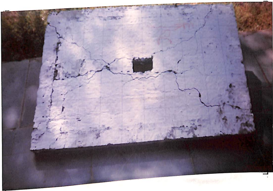
Fig.7.8 Crack pattern of Slab with 1% Central opening
