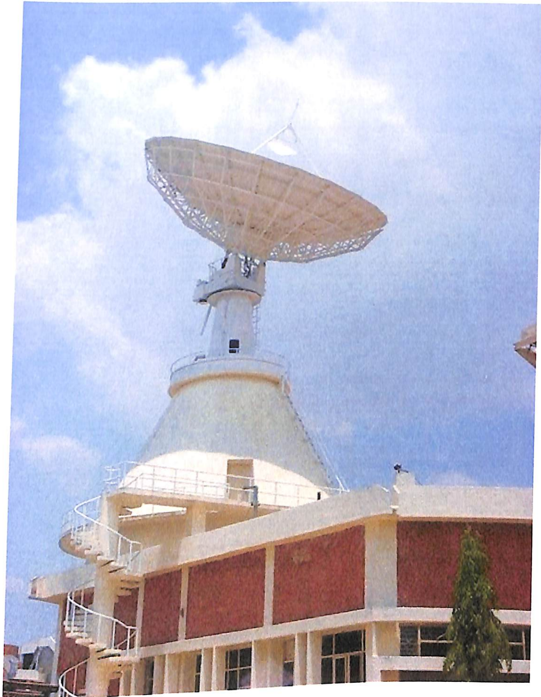
Fig. 5.3.1: Ext. C-band antenna (11 m dia)
